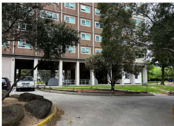
Figure 7. Ground floor undercroft of north-western corner tower.
