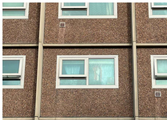
Figure 8. Detail view of fenestration.
