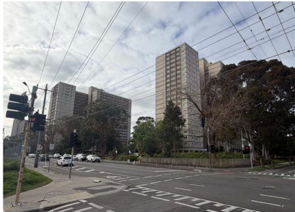
Figure 5. South-east facing view of towers fronting Elizabeth Street.
