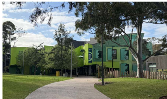
Figure 14. View of main North Richmond Community Health Centre building.
