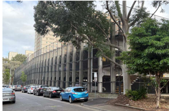
Figure 12. View of north-east Elizabeth and Church Street corner from Risley Street.
