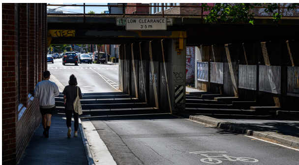
Image 23 - Balmain Street underpass
