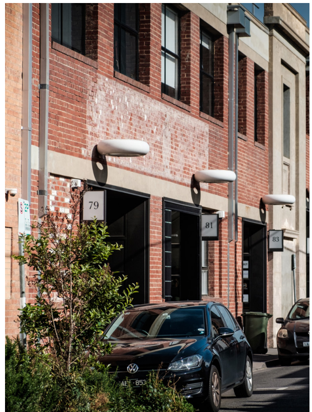
Image 10 - Warehouses converted to commercial tenancies
