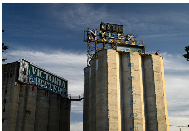
Image 16 - Nylex Sign and Silos at Richmond Maltings
