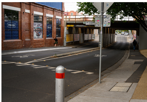
Image 25 - Balmain Street rail underpass
