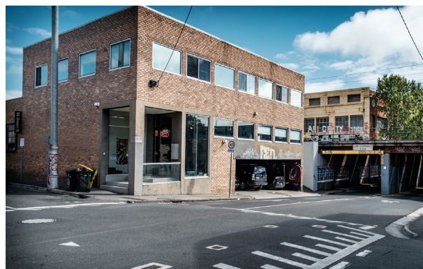
Image 77 - Balmain Street underpass looking west
