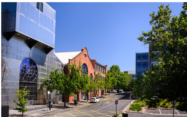
Image 71 - 658 Church Street - Former Power Station
