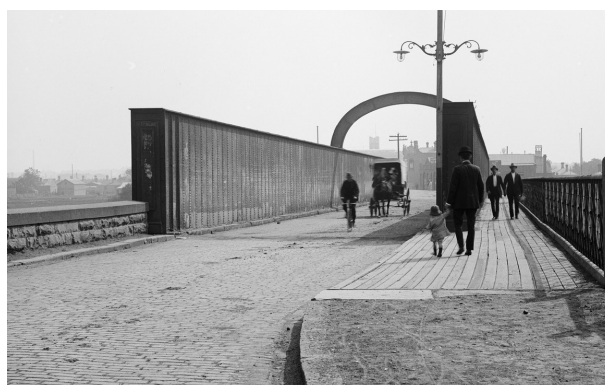
Image 4 - Church Street bridge (1914)
