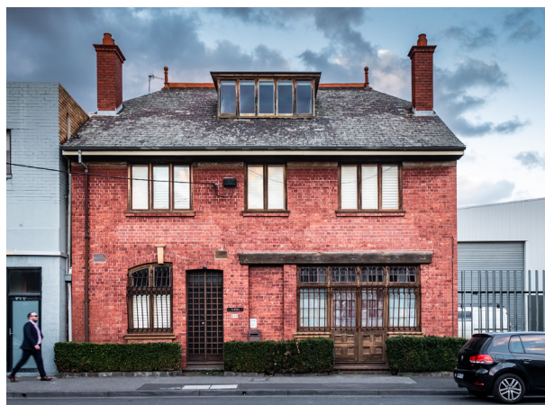
Image 76 - Former Yarra Hotel Cremorne Street
