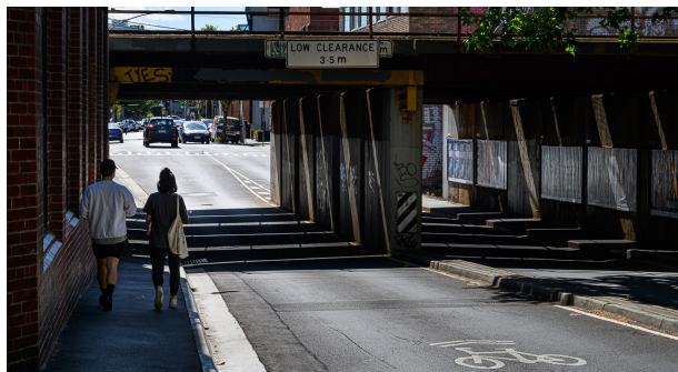
Image 23 - Balmain Street underpass
