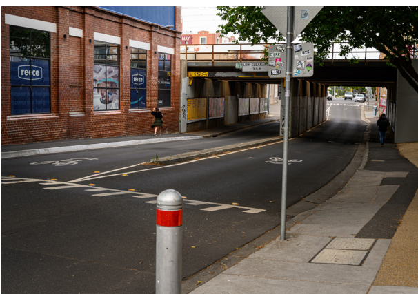
Image 25 - Balmain Street rail underpass
