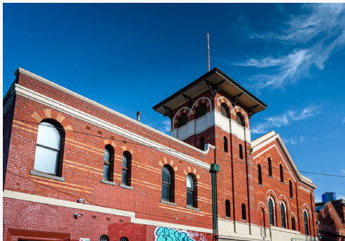
Image 65 - Former Richmond Power Station
