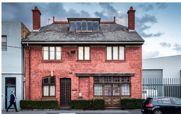
Image 67 - Former Yarra Hotel Cremorne Street
