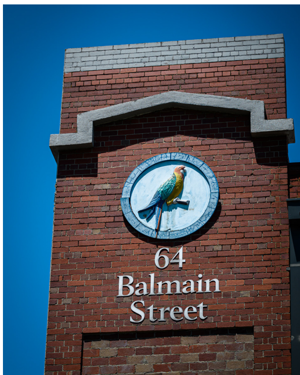
Image 85 - Rosella signage - Balmain Street
