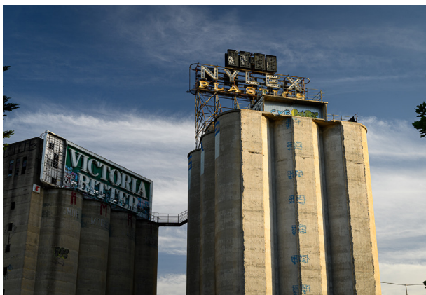
Image 16 - Nylex Sign and Silos at Richmond Maltings
