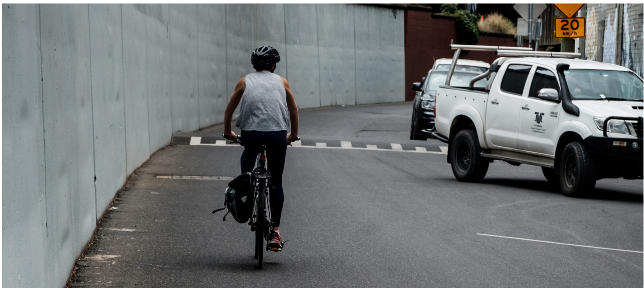
Image 27 - Shared road arrangement
