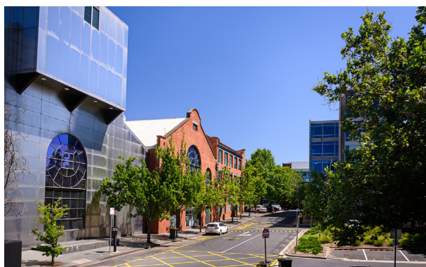
Image 71 - 658 Church Street - Former Power Station
