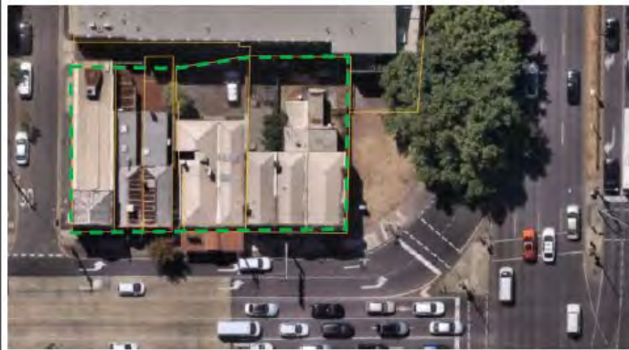
Figure 116. Current aerial photograph of 205-219 Victoria Parade (Source: nearmap, 14 February 2026)
