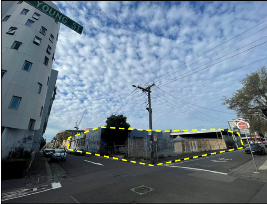
Figure 2: Subject site – Corner of Argyle and Young Streets (Officer Site visit, June 2026)
