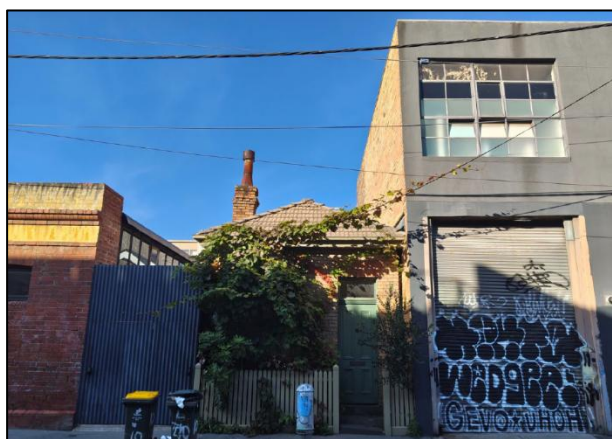
Figure 27 10 Argyle Street, rear of 260 Nicholson Street – street view
