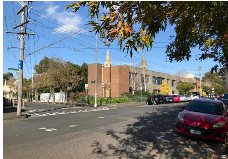
IMAGE 01 - EXISTING CLARKE ST POWER LINES
