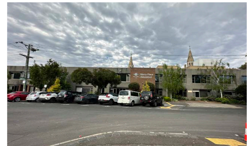
Site Investigation (CHT Architects)
