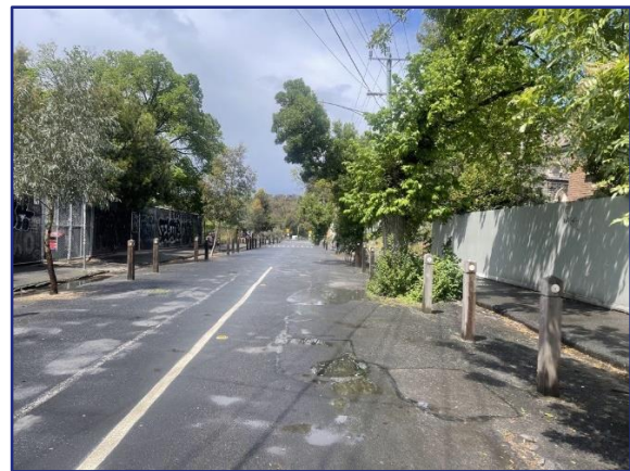
Figure 7: St Heliers Street - View East
