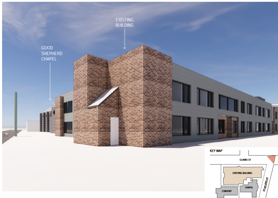
Figure 18 - Artist's impression of existing built form, looking south-east from corner of Clarke & St Heliers Streets
