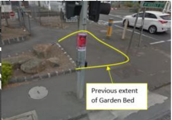
27) Removal of redundant infrastructure/barriers
