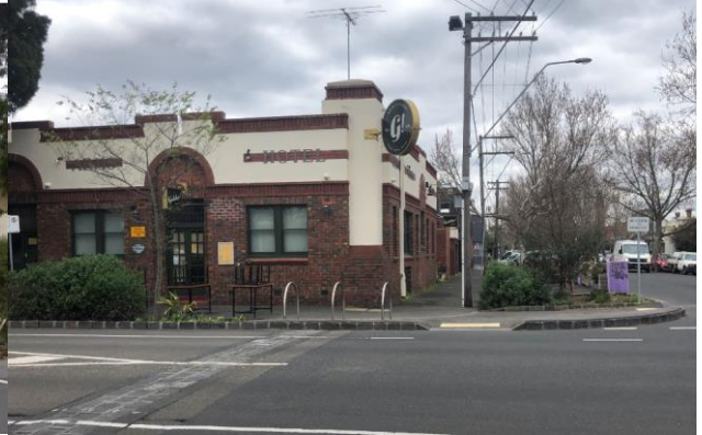
8) Kerb build out
