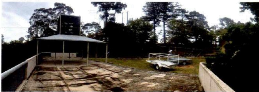
Figure 2: The side of the structure. (2018). Source: Yarra City Council.
