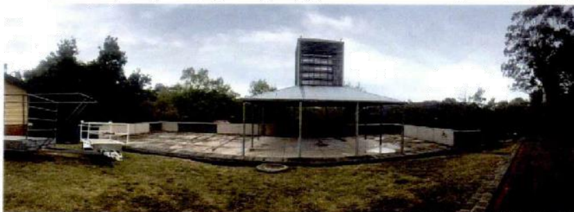
Figure 3: The side of the structure. (2018). Source: Yarra City Council.
