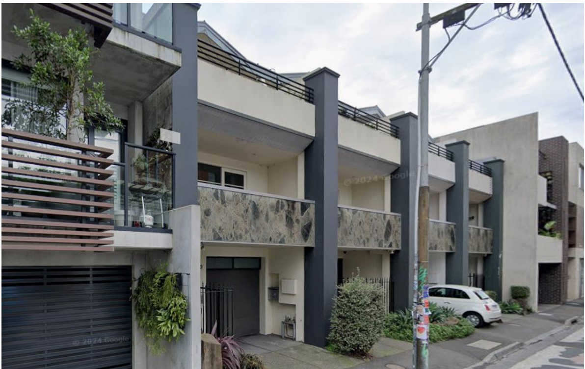
Dwellings to the north all have balcony areas.
