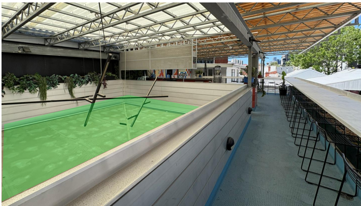
Behind the bar, the seating area wraps around. Highlighted in green is a tarp/screen system, which separates the first-floor and ground floor areas. This essentially means that noise generated on the ground floor has potential to propagate up and out of venue, into the first floor area.
