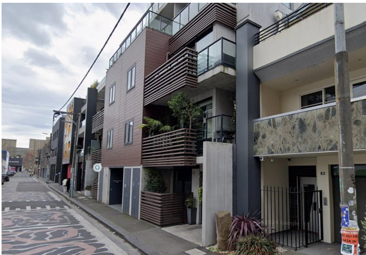
Dwellings to the north all have balcony areas.
