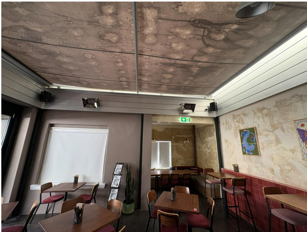
On the ground level, we can see the tarp/screen from below.
