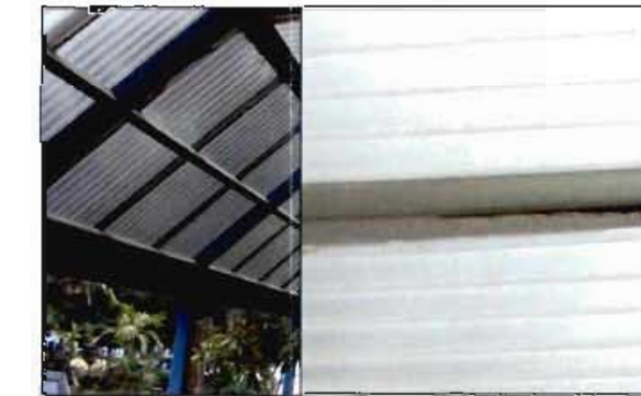
RT-01 AMPELITE WONDERGLAS GC IN OPAL HARDIES SUPER 6 PROFILE
