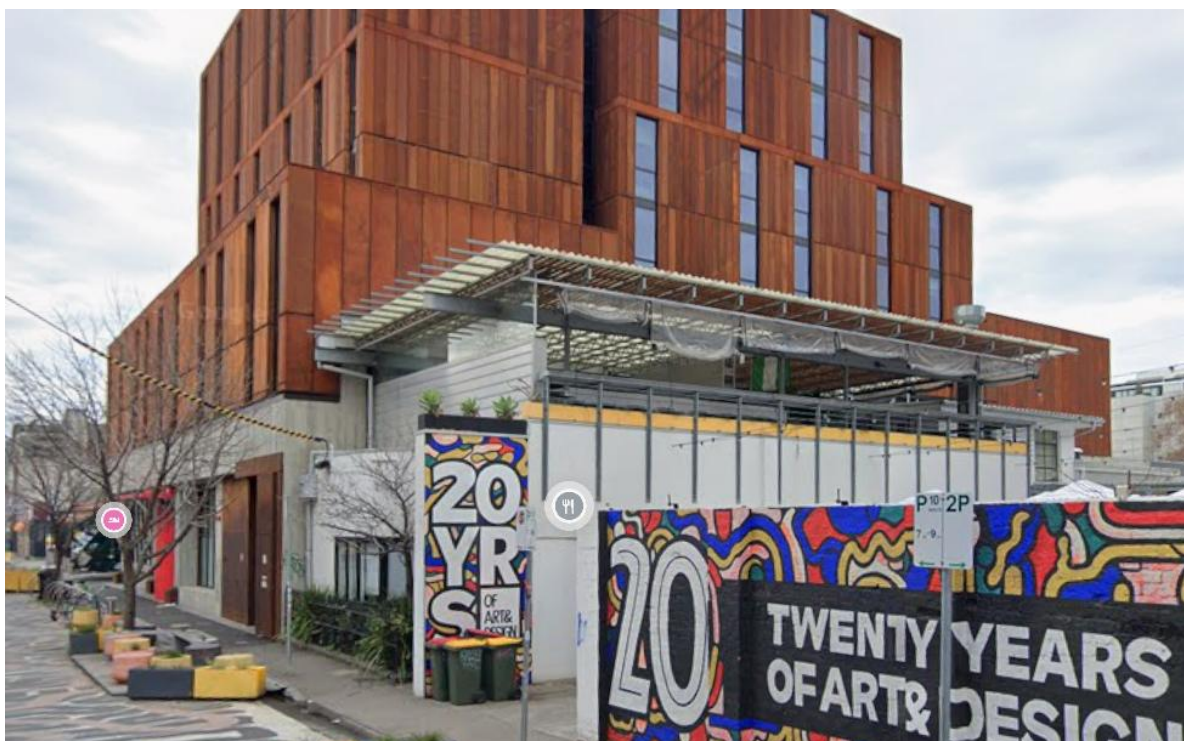
To the east, a hotel. There are no balconies overlooking the roof system.
