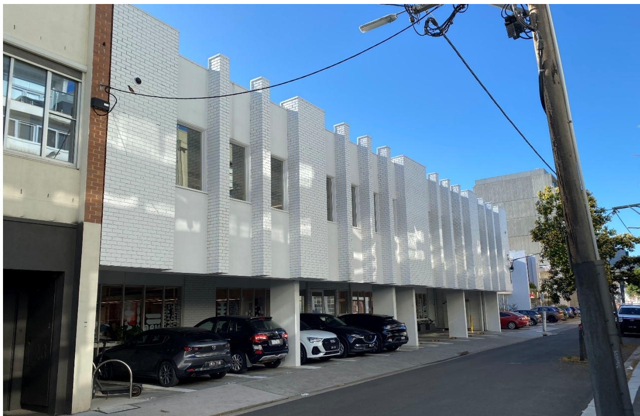
Figure 1 - Viewing southeast along Wangaratta Street to front of No. 31-43 Wangaratta Street. Source: Officer site visit 6 November 2025
