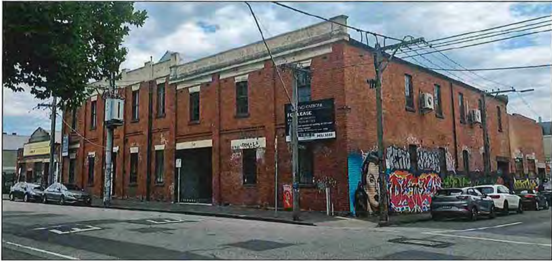
15 to 17 Kerr Street
