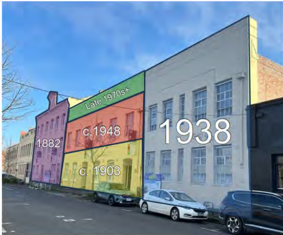
Figure 1 - Extract from Heritage memorandum prepared by Bryce Roworth (February 2025) showing annotated view of the different periods of construction of the Victoria Street facade.
