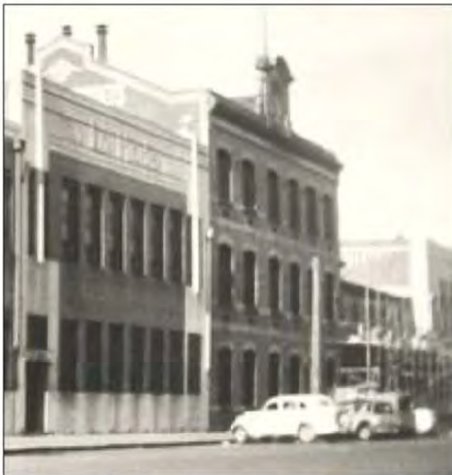
1948 view showing scaffolding in front of the intermediate structure between the 3 storey former Acme factory (centre) & the 1938 addition (far right), with the central first floor possibly under construction.
