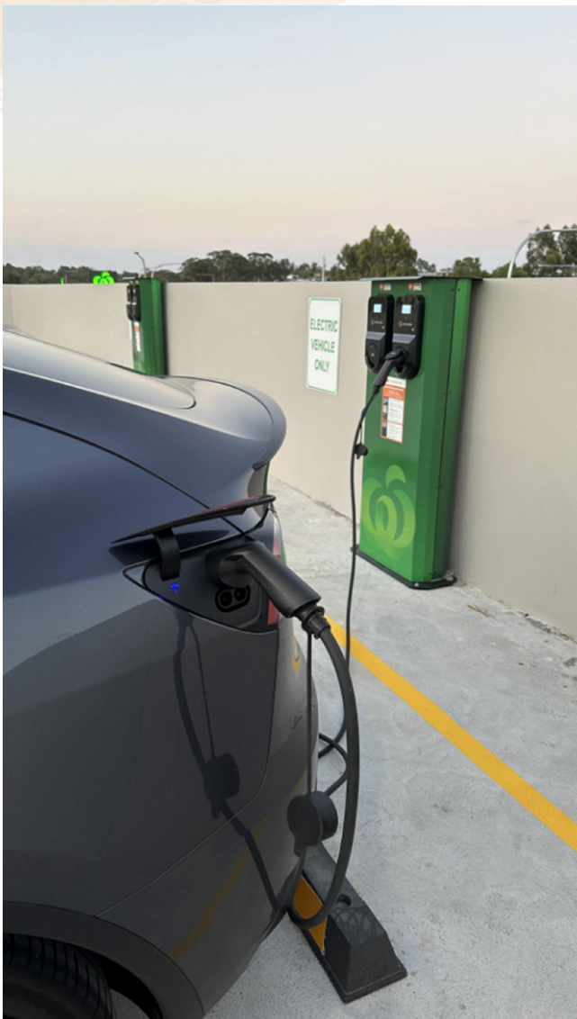
Figure 4 EV charging for businesses
