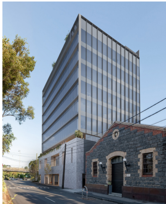
Figure 7: Render of the development from west along Madden Grove (Studio McCue March 2025)
