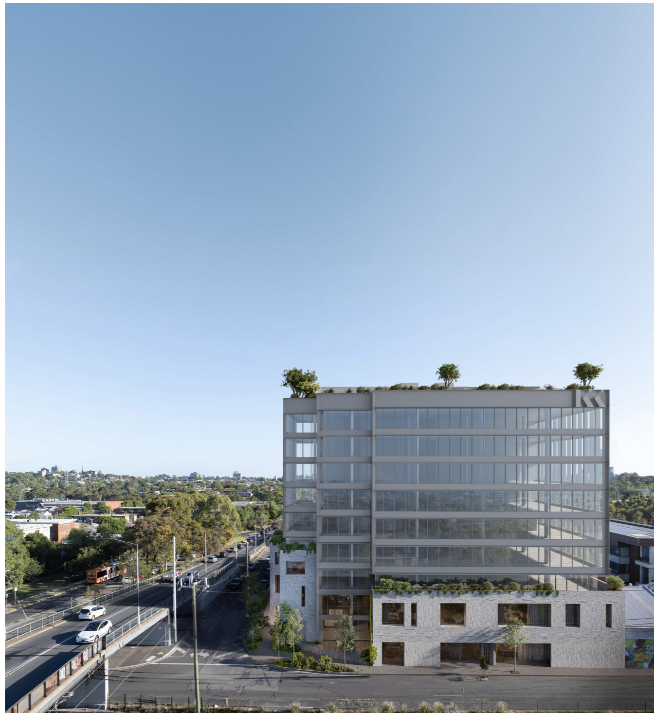
The indented corner to the north-western podium form respects the setback to the Dutton's Garage building with a strong datum of the brick podium contextually relevant to its neighbours.
