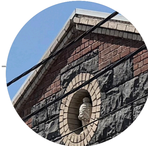
EXTENSIVE USE OF MASONRY AT STREET LEVEL INFORMS THE SELECTION OF PUNCHED BRICK OPENINGS TO THE PODIUM FORM
