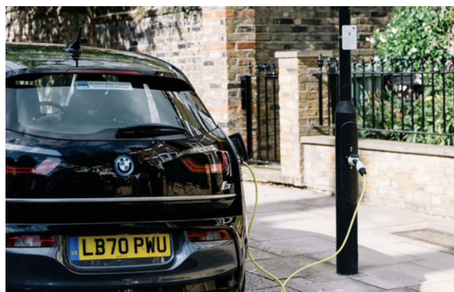
Figure 15 Typical London lamp post kerbside charging
