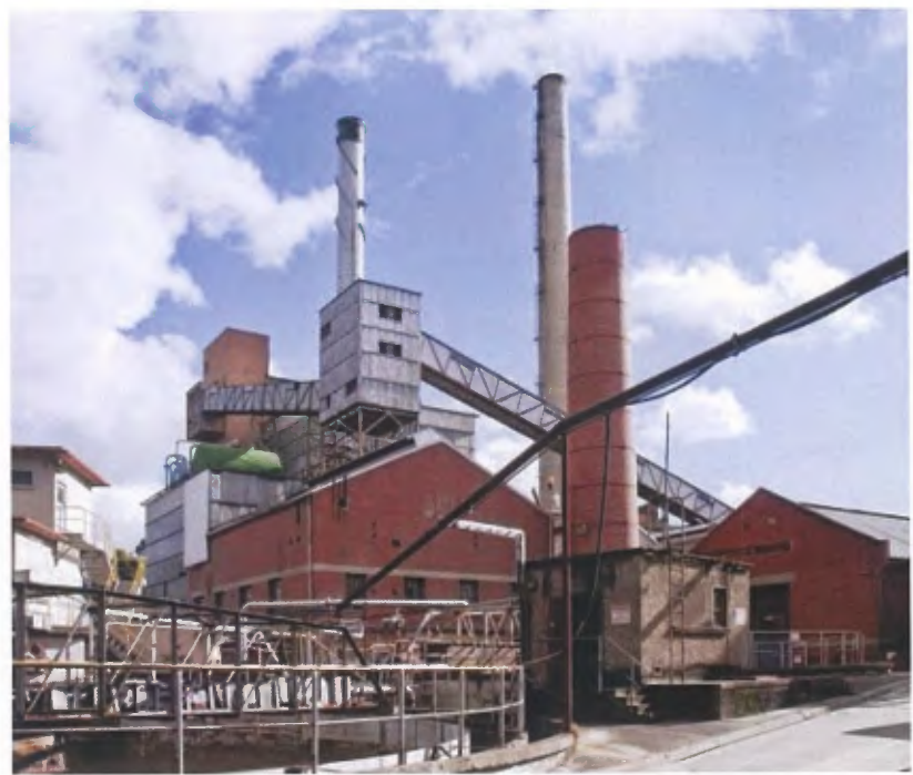
VIEW TOWARDS c.1920 BOILER HOUSE, WITH c.1954 BOILER HOUSE AT REAR
