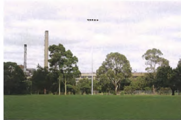
9 The 1954 Boiler House viewed across Alphington Park.
