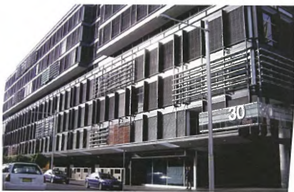
MULTIPLE FACADE SHADING AND RECESSED MASSING DETAILS (30 The Bond, Sydney - Lend Lease design)
