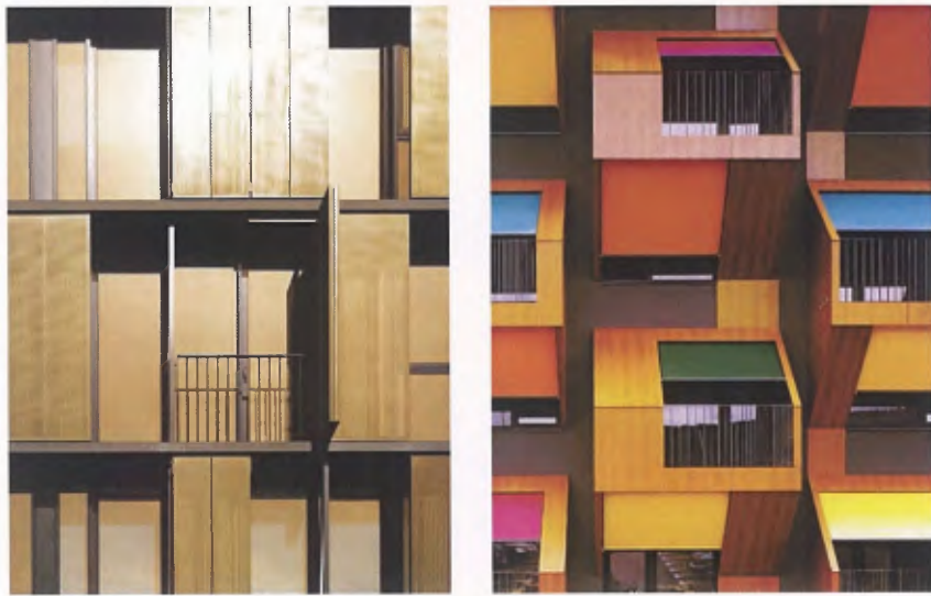
APARTMENT BALCONIES AND SCREENING
