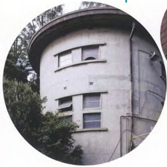
RIVER PUMP HOUSE
