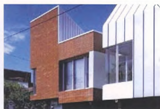
BRICK ENDS (Napier Street Housing - Kerstin Thompson Architects)
