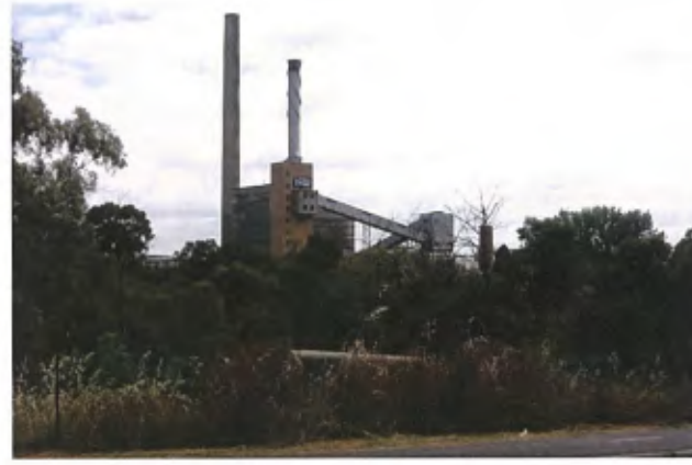
7 The 1954 Boiler House viewed from Yarra Boulevard.
