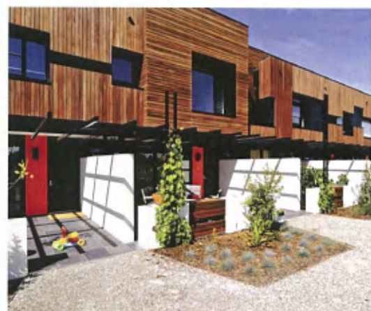
TOWNHOUSE ARTICULATION THROUGH FENESTRATION (Heller Street Brunswick - Six Degrees Architects)
