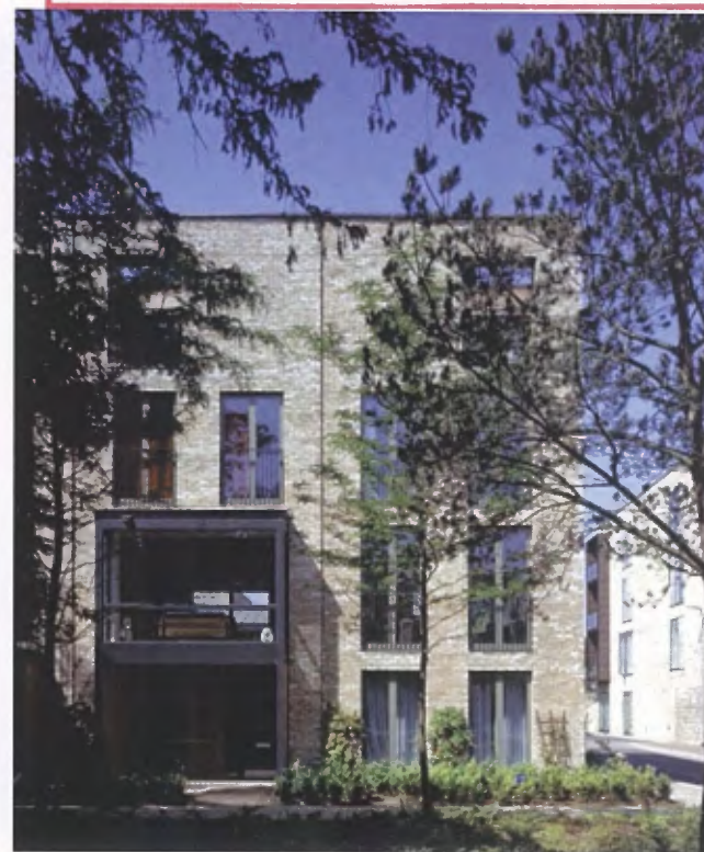
CLEAR ENTRY DEFINITION (Accordia Cambridge - Feilden Clegg Bradley Studios)
