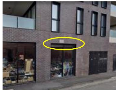
Figure 3: Ventilation louvres – external view
