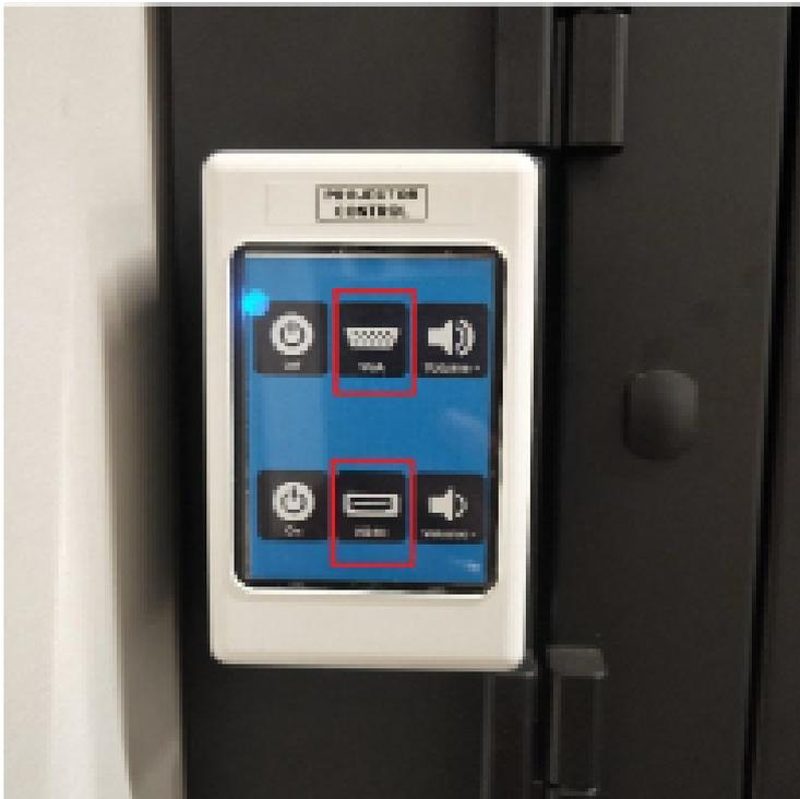
7. Locate the small input selector box, directly on top of the audio control panel
