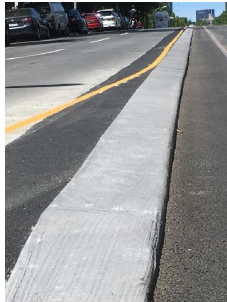
Figure 13: Combined barrier and semi-mountable kerb installed in Lygon Street in 2018
