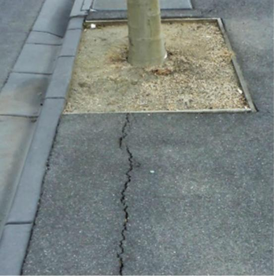
A tree is planted in a tree pit with a metal grate. The asphalt surface around the pit is cracked, indicating poor maintenance. |
