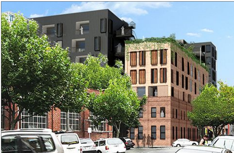
Figure 20 Illustration of approved development currently under construction at 221 Kerr Street, Fitzroy (individually significant in HO334). Two storey heritage building, 6 additional levels approved with a setback to the level above the heritage facade to create a shadowline, no setbacks to the two levels above, greater partial setbacks to the remaining levels.
