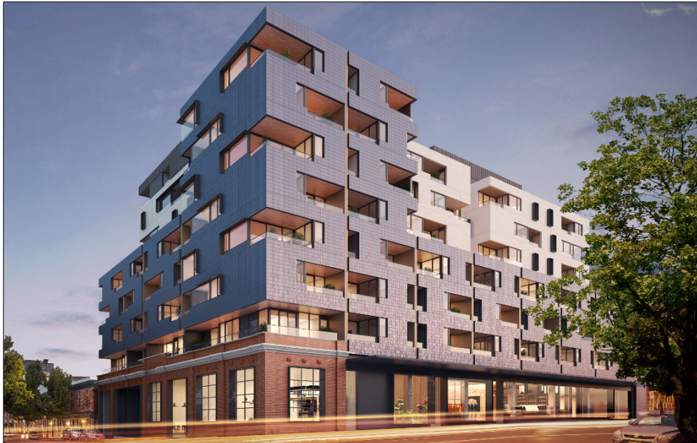
Figure 15 Illustration of the development currently under construction at 239-245 Johnston Street, Fitzroy (Contributory in the South Fitzroy Precinct, HO344). Single storey heritage building, 9 additional levels with a setback at first floor to create a shadowline, and no setback from the heritage facade at the second floor and above.
