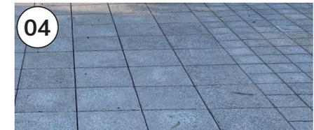
04 Precast concrete paving with basalt aggregate
