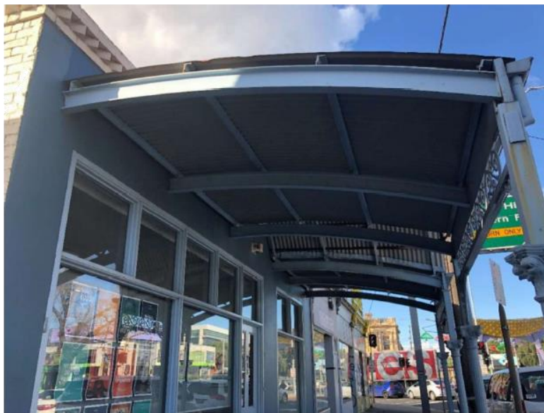
Figure 7. Looking east to the canopy at 211-213, showing later steel structure above cast iron verandah posts.
