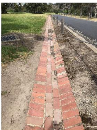
2019, S facing image showing a spoon drain comprised of potential re-used bricks.
