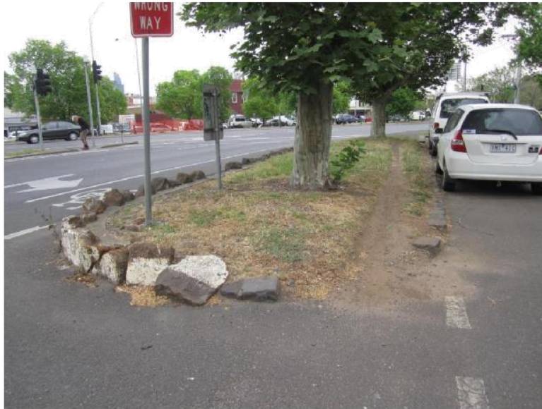
Figure 11: Westernmost median adjacent to the Alexandra Parade intersection. Uncut basalt blocks remain relatively intact to the central traffic lanes, with the border to the service lane comprised of standard cut basalt blocks.
