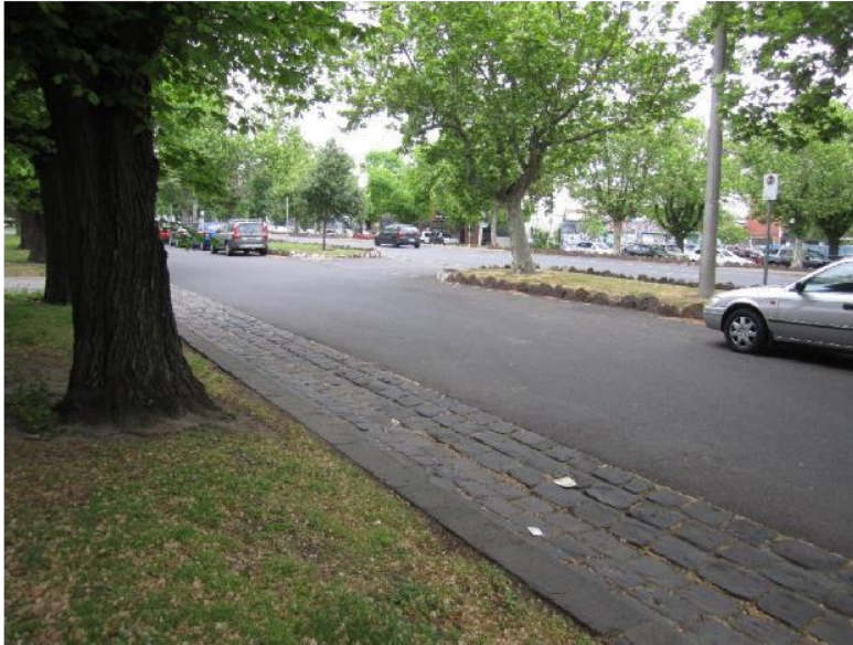
Figure 13: Type 3 curb and drainage channel.
