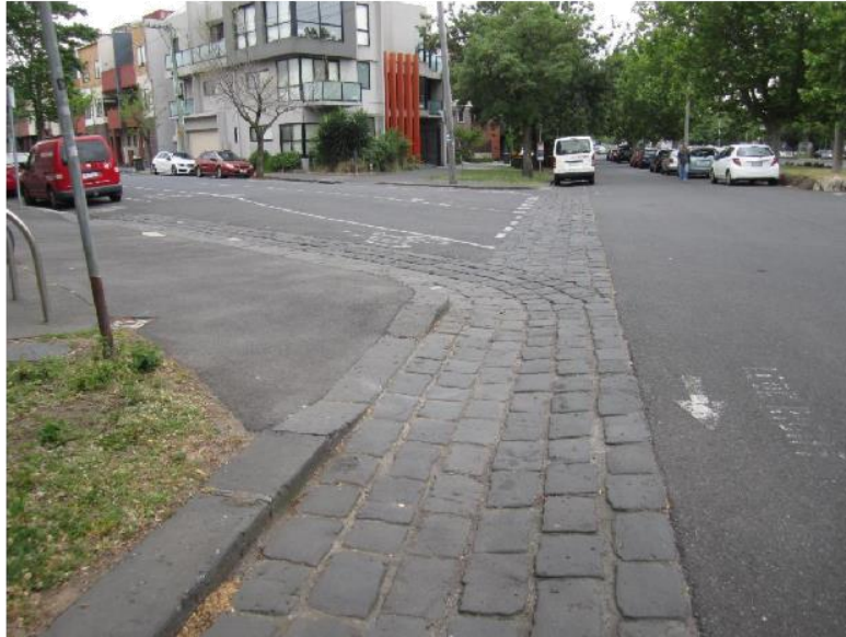
Figure 19: Northern drainage channel configuration of six rows of basalt pitchers continues across the intersection of Napier Street and the Queens Parade service lane, terminating at the intersection with Jamieson Street.
