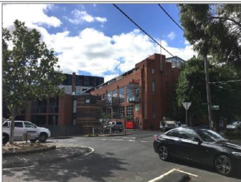
Byfas Ltd Factory – 8-16 Trenerry Crescent, Abbotsford (HO314 – Yarra Falls Precinct) *Note: land surrounding the art deco building is not within the HO
