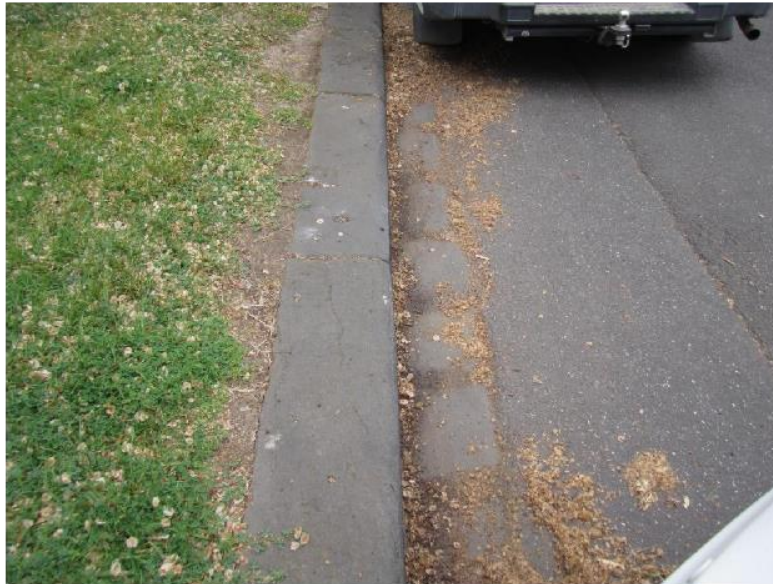
Figure 12: Type 2 curb and drainage channel.
