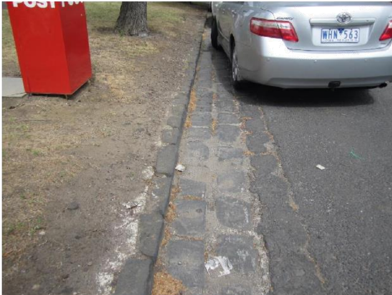
Figure 16: Type 6 curb and drainage channel.
