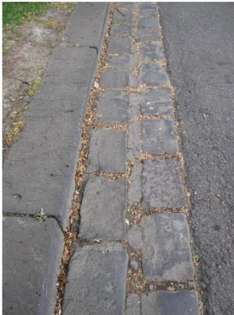
Figure 14: Type 4 curb and drainage channel.
