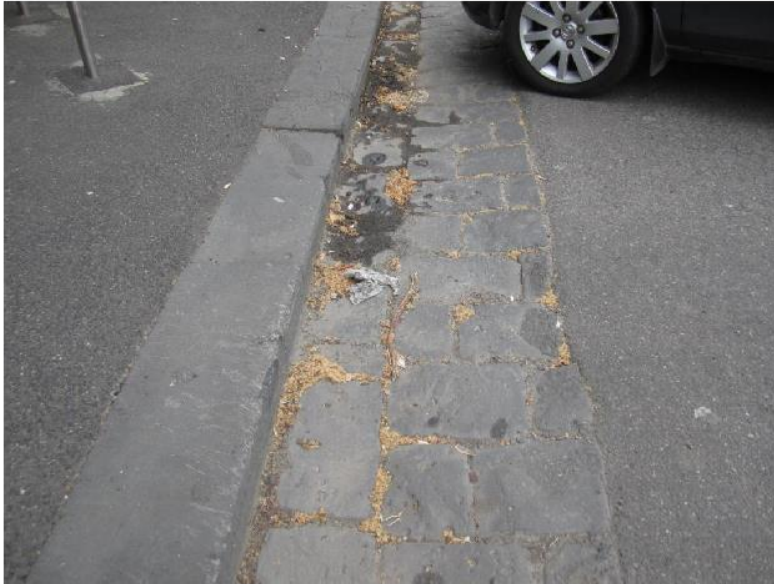
Figure 15: Type 5 curb and drainage channel.
