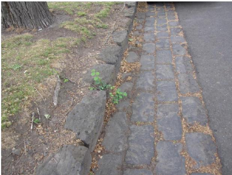
Figure 18: Type 8 curb and drainage channel.
