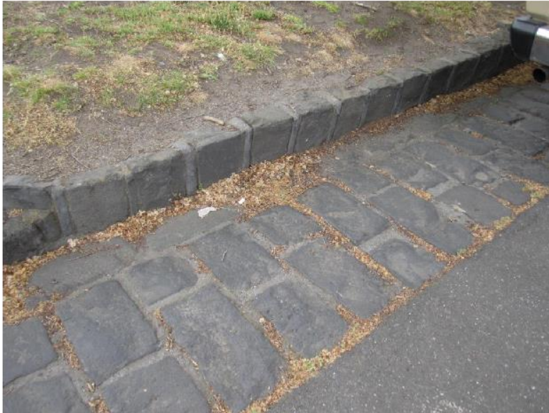
Figure 17: Type 7 curb and drainage channel.
