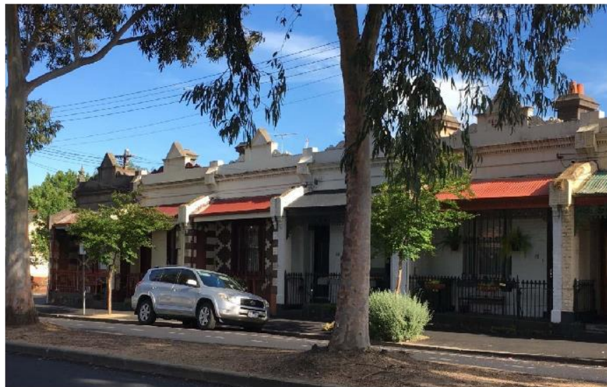
Figure 4. North Carlton (row of small terraces with minimal street setbacks).
