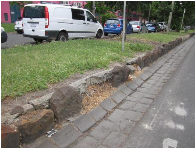
Figure 10: Median between Alexandra Parade and Napier Street. View of missing uncut basalt blocks and basalt pitcher drainage channel.
