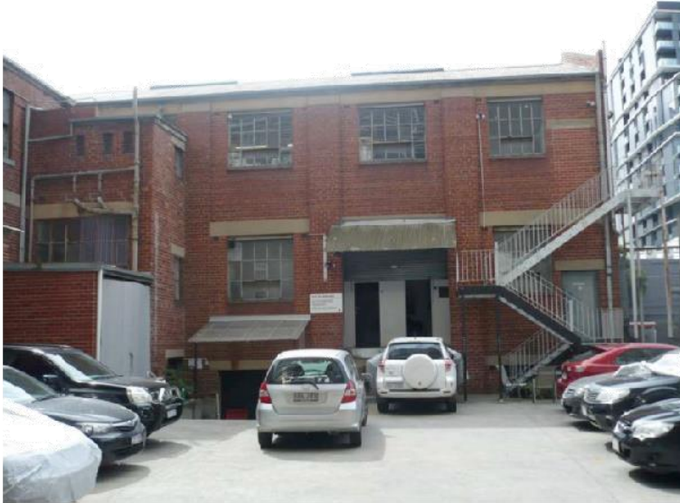
Figure 3: The section of the car park to the right of this photo forms part of 14 Glasgow Street that is within HO109
