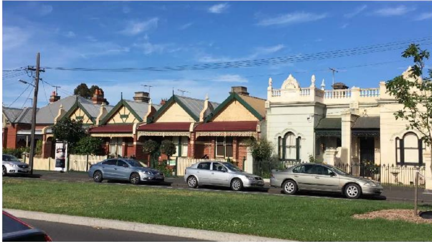
Figure 8. North Carlton (row of mixed terraces, single fronted but with more generous frontage and front setbacks, wide open street setting).
