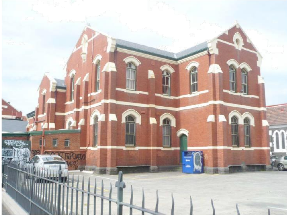
1897 school. The single storey hall section is behind.
