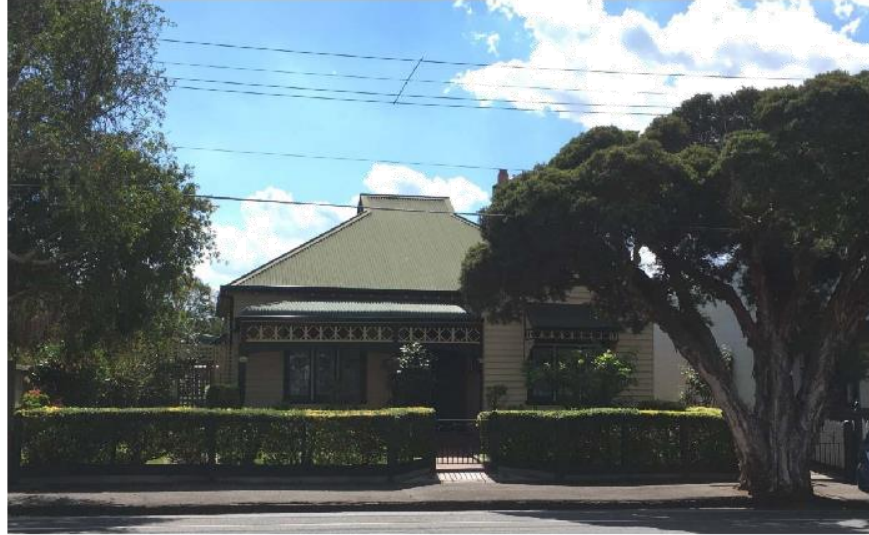
Figure 10. Clifton Hill (wide generous garden block, open wide street, large detached house).
