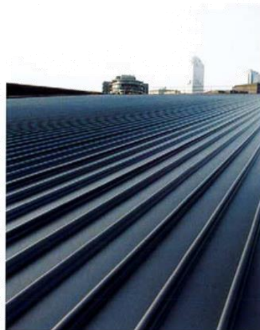
MR-1 METAL ROOFING Metal Roofing Finish: Zincalume
