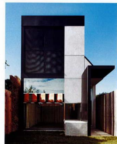
ME-1 PERFORATED MESH Perforated Mesh Opening: Max. 25% transparency
