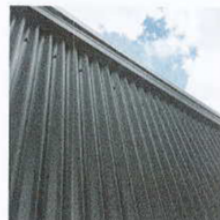
EXISTING CANOPY ROOF: EXISTING CANOPY ROOF TO BE REPLACE WITH NEW CUSTOM ORB ROOF SHEETS. COLOUR: DARK GREY
