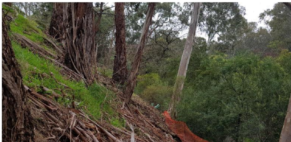
Figure 9: Planted trees on embankment - Trees on the embankment are 20+ year old non-indigenous natives. The trees on the embankment are growing at different angles to each other. Investigate for slumping or ground heaving to determine stability of the trees.
