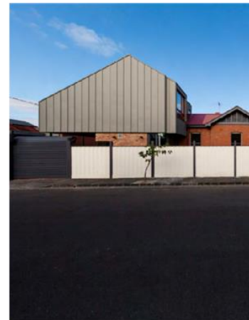
STANDING SEAM CLADDING & ROOF
