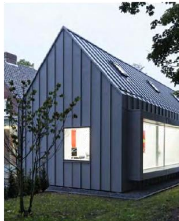
STANDING SEAM CLADDING & ROOF
