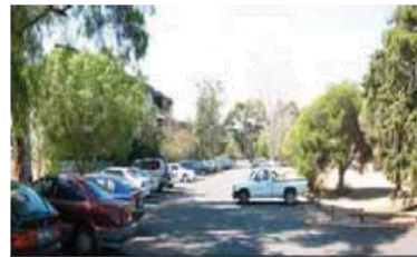
Photo 9: Asphalt Surface Main Car park
