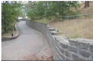
Photo 12: Staggered Bluestone Retaining Wall
