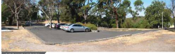
Asphalt carpark outside toilets
