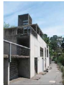
Photo 5: Concrete Storage / Change Room Building
