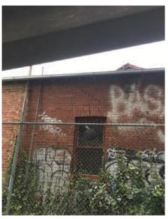
Photo 6: North Wall looking externally. Re-constructed where ivy had penetrated brick courses, Large crack right through lintel & reflective cracks right along north wall.
