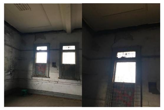
Photo 12: South-West corner of Room 9 (Hall). Crack to west wall not repaired, internally. Crack looks to have got larger compared to the photos in previous
