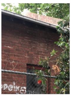
Photo 7: North wall has new formation of cracking above lintel, cracks are new and was not observed and documented in previous report.
