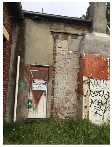
Photo 15: Rear Exit at east end of main entry hall. Disconnected downpipe and heavy water damage to external render. Single story toilet block has been demolished and external brickwork exposed which is heavily cracked.
