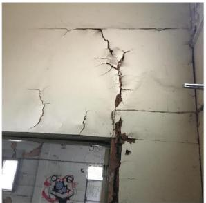
Photo 23: Large cracks & rotting of timber walls from settlement movement and water damage. Crack was observed at entrance of room 8 & 6.
