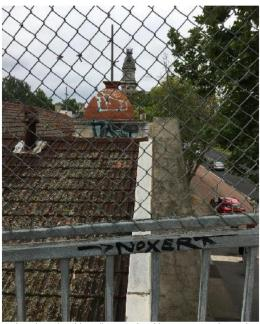
Photo 2: Turret structure above main entry. North and South gable walls warped and leaning outwards. By observation current state looks similar to previous report photos.
