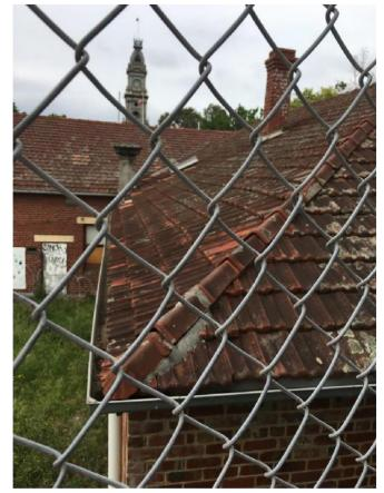
Photo 5: Tiled roof at North-East corner. Tiles to be removed, repaired and re-pointed. Eaves, gutters and downpipes to be replaced.
