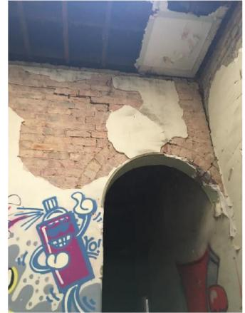
Photo 20: Internal arch leading from room 8 to 7, crack looks to have got worse since previous report.
