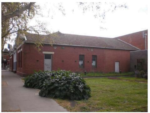
Photo 14: South wall of hall. Two number tie backs at line of internal engaged piers. Wall at east re-constructed.
