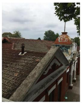
Photo 3: Main roof viewed from North-West. Remove tiles, re-level battens and re-instate tiles, central part of roof looks bowed which was also stated in previous report.
