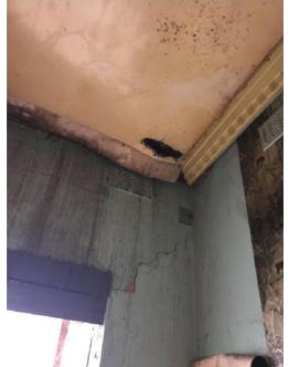
Photo 24: Room 12, first floor at corner of south east wall, cracks starting to form, and roof is starting to fall down from heavy water damage. Walls are heavily water damaged also with large amounts of rot.
