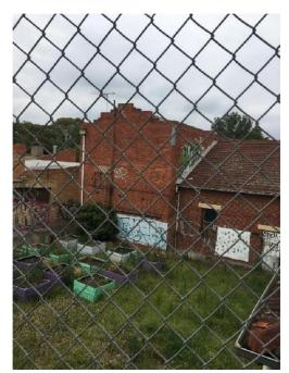
Photo 4: Existing tiled roof viewed from pedestrian footbridge, Timber caretakers & timber toilets have been demolished since previous report photos.
