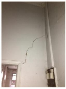
Photo 17: Other side of wall shown in photo 16, crack is on both faces of internal brick work wall.
