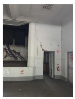
Photo 16: Cracking above door (leading from Hall (9) to Room 10A, cracking looks to not have gotten worse since previous report.
