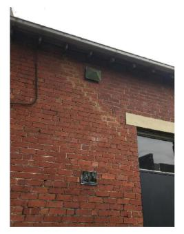
Photo 10: South-West corner of Hall. Foundation may have dropped. Wall repaired previously, in buildings current observation repair is starting to crack again at top of brick wall.
