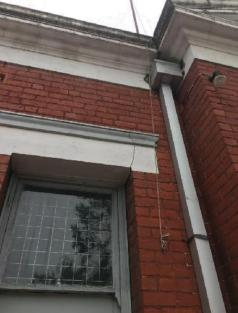
Photo 21: Front Façade West Wall (Hoddle St) has a large crack through lintel at support where lintel is bearing on brickwork. Was not observed and documented in previous report.
