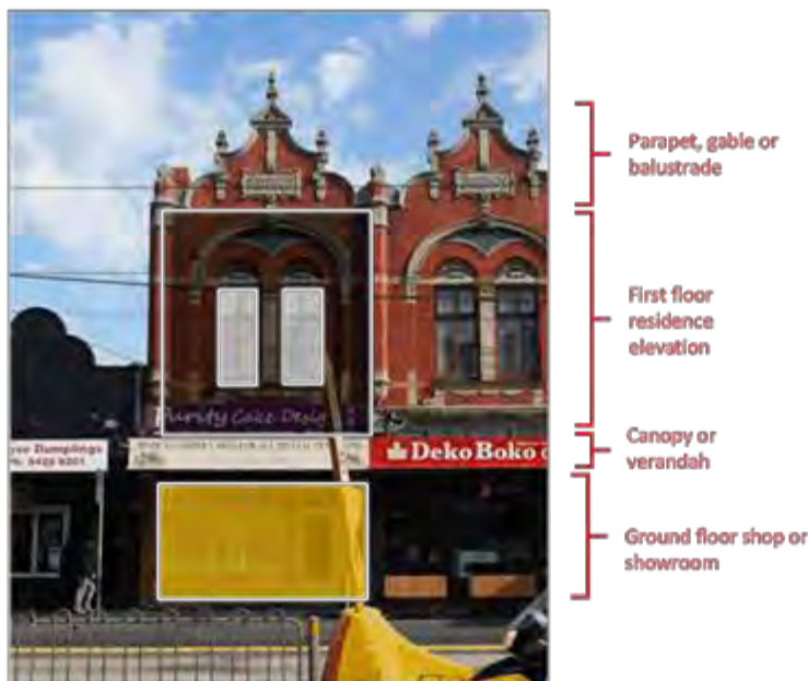
Figure 12. Two-storey shop/residence showing the typical relationship between solid (walls) and void (windows) on the front façade. The grey shaded area is the first-floor façade wall with light grey shaded windows making up less than 40% of the wall area parapet (excluding the parapet, gable or balustrade), and the yellow shaded shopfront glazing and entrance door occupies the majority of the ground floor façade.
