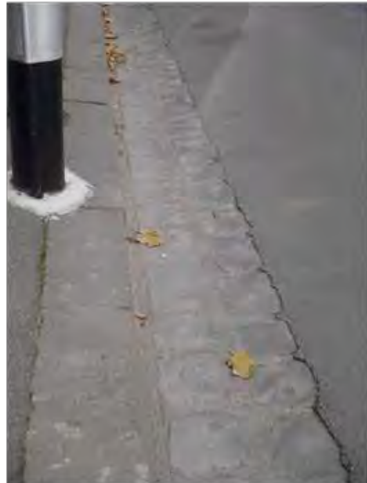
Figure 5.12 : View south showing the bluestone kerb and channel along the east side of Nicholson Street. The channel is approximately 500 mm into the road. A similar channel is present on both sides of Gertrude Street.
