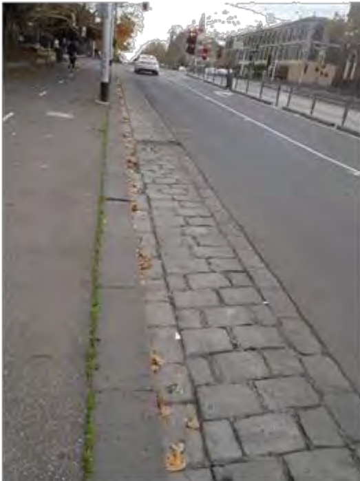
Figure 5.11 : View north showing the bluestone kerb and channel along the west side of Nicholson Street. The channel is approximately one metre into the road.
