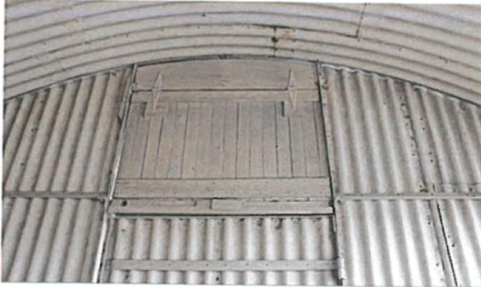
Figure 7 Detail of opening & door, east elevation. Note original timber infill above the opening.
