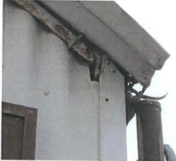
Figure 8 Detail of typical damage, west elevation.
