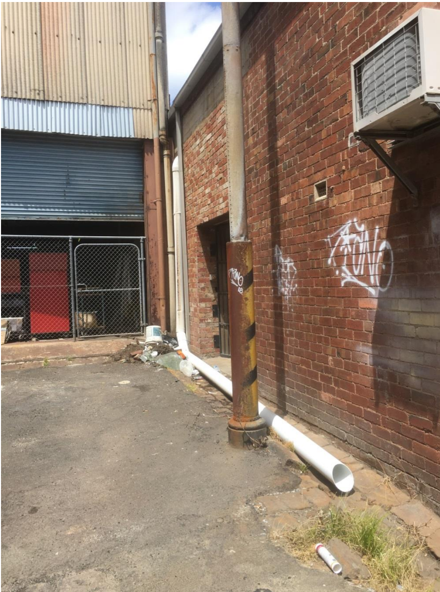
One of the existing Legal Points of Discharge for the Site. For new building, the roof drainage must be connected to an underground drain (to be provided by the developer).
