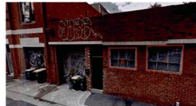
6. Screened Window 7. Screened Window
