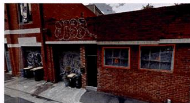
6. Screened Window 7. Screened Window
