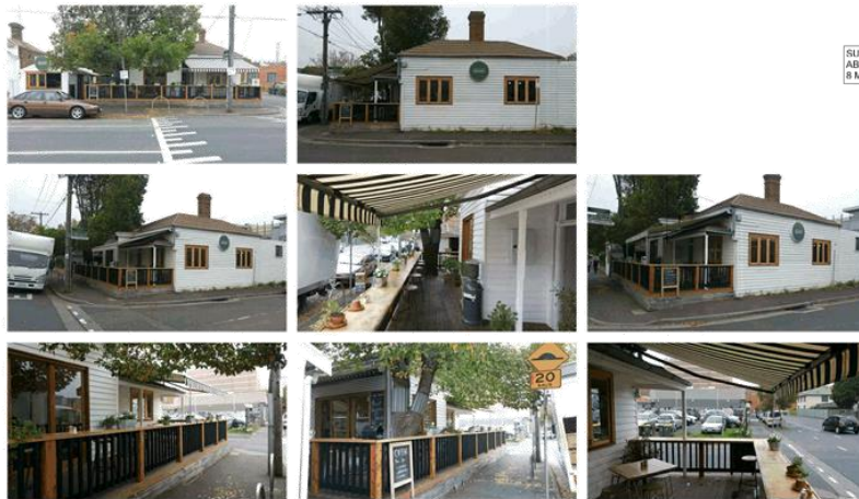
2 EXISTING CONDITION PHOTOS A.0.00
