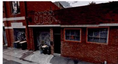
6. Screened Window 7. Screened Window
