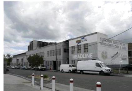
Factory on east side of Emma Street, looking south.
