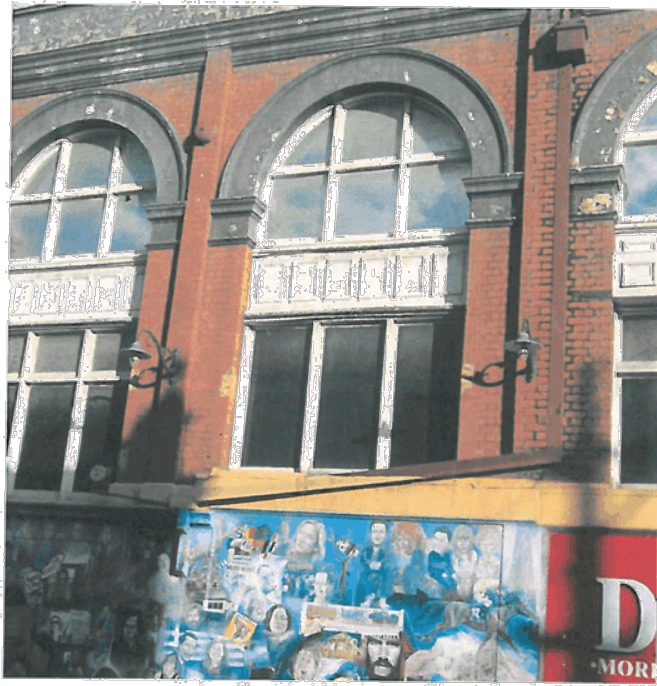
Image of light fittings to Green Street elevation, prior to removal for conservation works.
