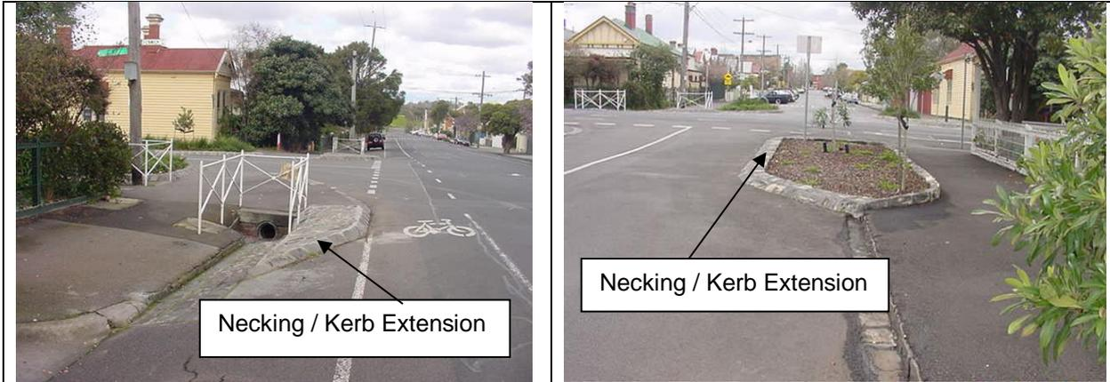
Typical necking/kerb extension in residential areas where the necking kerb has been constructed to match the street bluestone kerb and channel.
