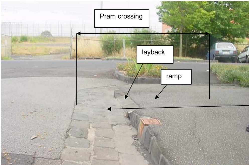
When bluestone pitcher channels at pram crossings are reconstructed the pitchers in front of the pram crossing will be cut in half and laid smooth side up.
