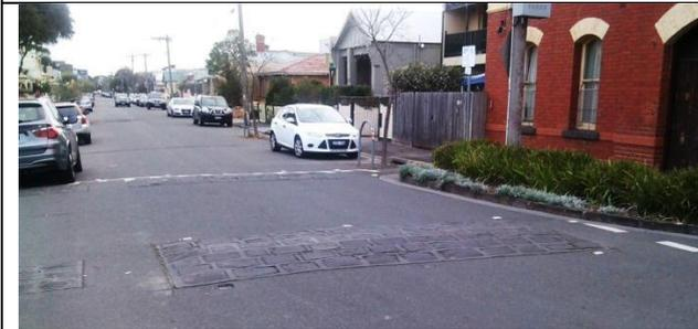
Bluestone road hump. When reconstruction occurs the road hump will be reconstructed in asphalt.
