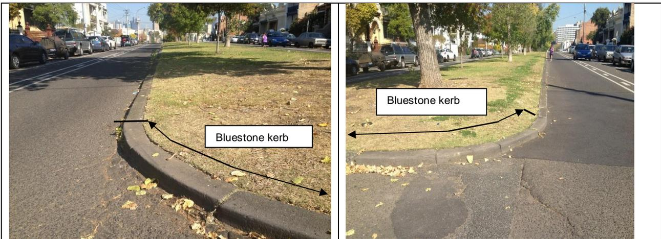
Medians historically constructed with precast concrete kerbing in North Carlton. Where the existing precast concrete end radials are damaged they will be replaced with concrete. If the end radials are bluestone, they will be replaced with bluestone.
