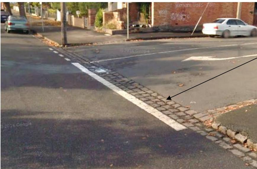
A wet crossing with a one or two pitcher wide layback. This will be built where there are no existing bluestones in the ramp or pedestrian
