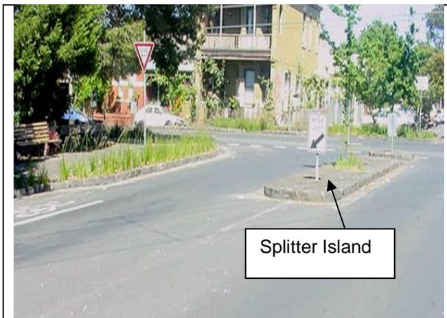
Splitter island constructed with bluestone to match with the street bluestone kerb and channel in a residential area.
