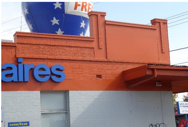
Yarralea Street (east) elevation – parapet detailing
