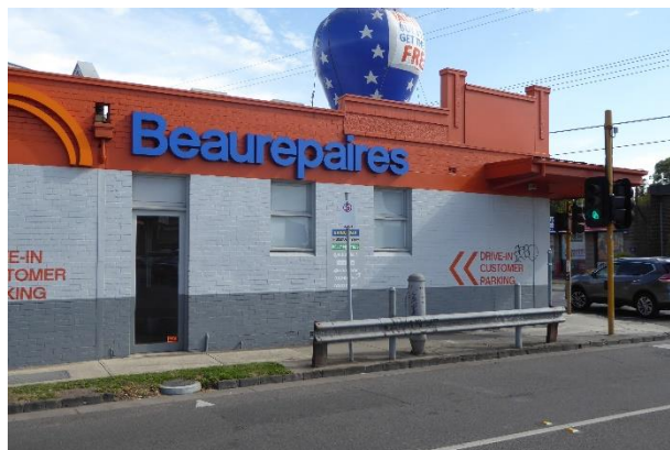
Yarralea Street (east) elevation
