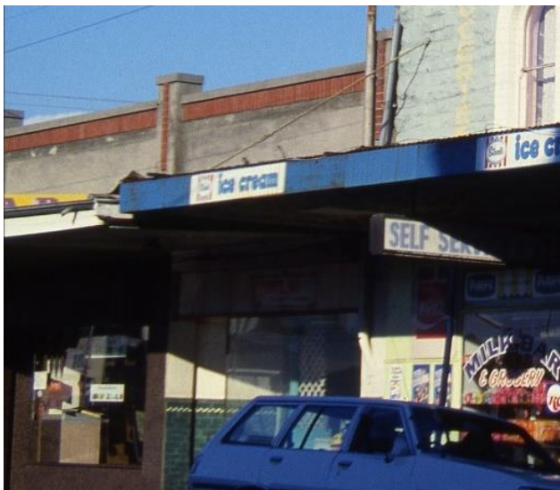
Photograph dated 1982 showing original presentation of parapets (Source: Darebin Archives LHRN3652)
