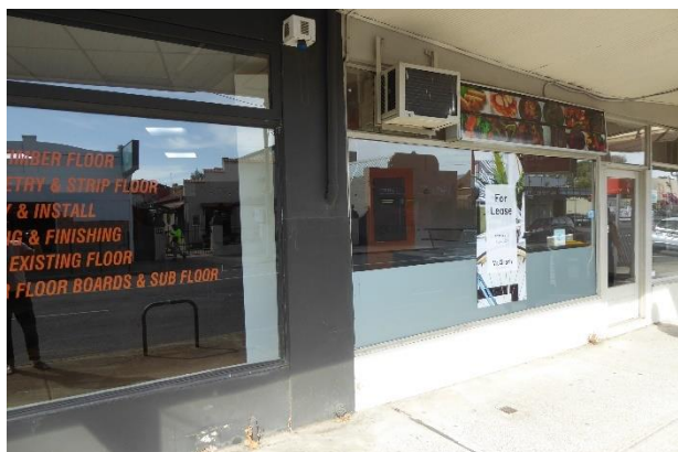
Nos 732-734 Heidelberg Road - shopfronts
