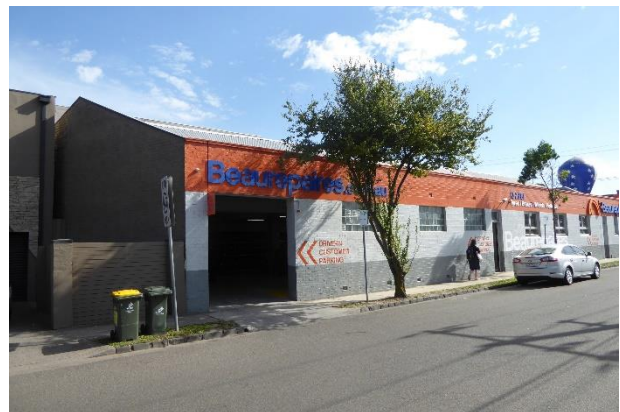
Yarralea Street (east) elevation
