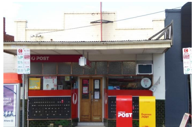
730 Heidelberg Road – parapet and shopfront
