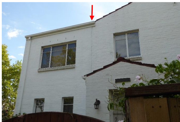
House – Park Crescent (primary) façade Junction between original (right) and additions (left)
