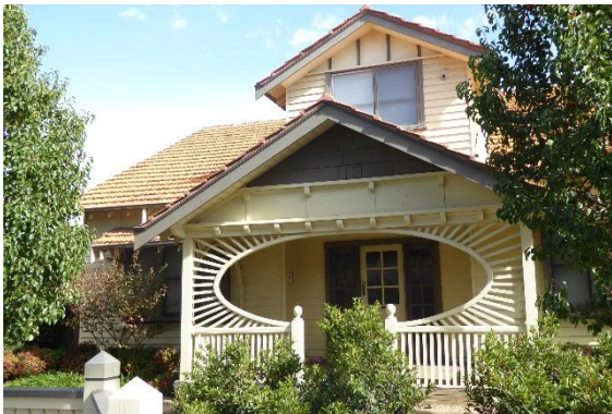
59 Yarralea Street – east elevation, included in HO362
