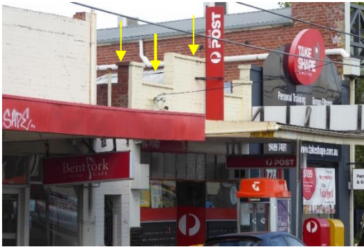
No. 730 – the original parapet, east return and hipped roof are visible from Heidelberg Road
