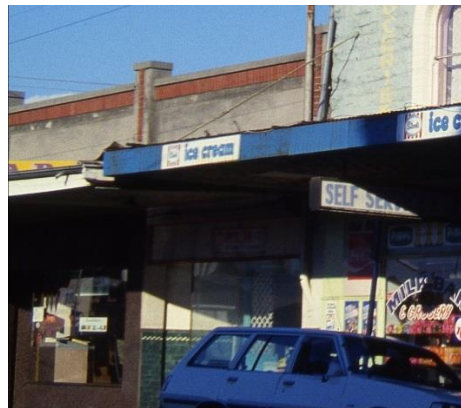
1982 image – showing original parapet detailing
