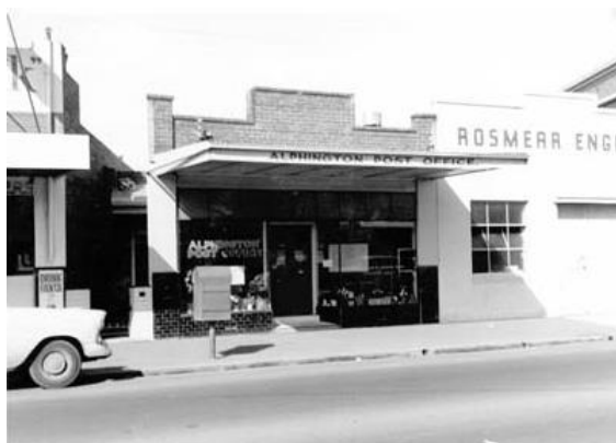
1968 Heidelberg Road elevation – no. 730 (Alphington Post Office) (Source: NAA)
