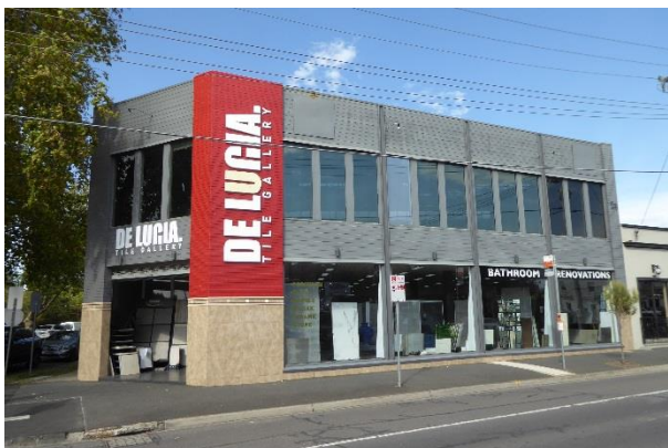
Heidelberg Road (north) elevation
