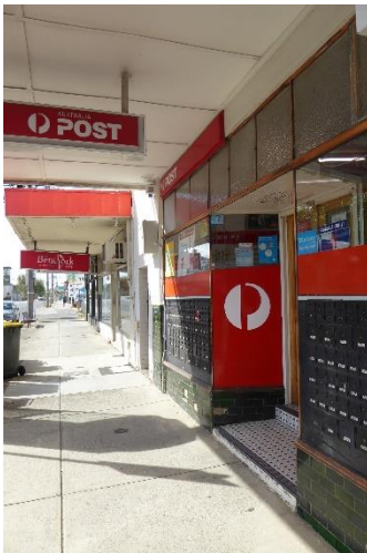
No. 730 – original shopfront
