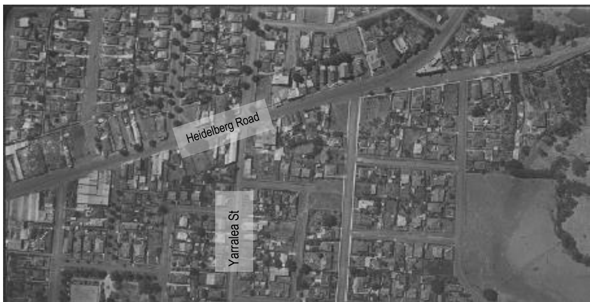
1945 Aerial, Heidelberg Road – east end of study area (between Parkview Road and Lucerne Crescent) The northern half of Alphington East Precinct (HO362) is evident (Source: Landata)
