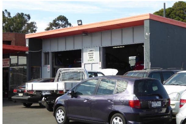
Heidelberg Road - west wing
