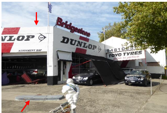
Heidelberg Road – original parapet roof, openings, doors and windows of tyre outlet. Original bowser pipes to front of site (indicated).
