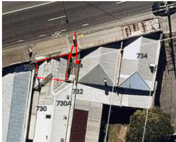
No. 730 – original section of roof visible from Heidelberg Road indicated by the dotted line. Visible parapet returns of nos 730 and 732 indicated by the red arrows (Source: Nearmap)
