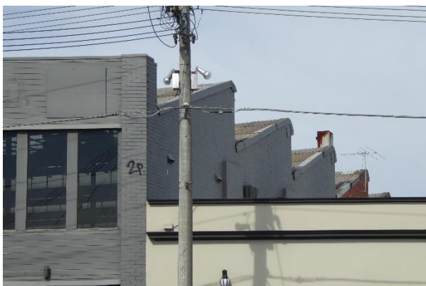
Sawtooth roof forms from Heidelberg Road
