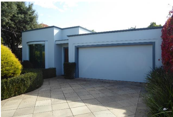
2 Killop Street – façade/south elevation, included in HO362
