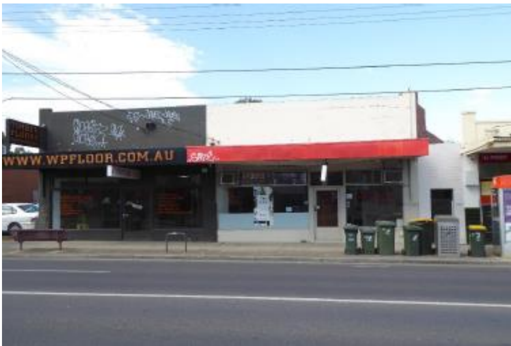
Figure 2: 730A (right), 732 (Centre) and 734 (left) Heidelberg Road, Alphington
