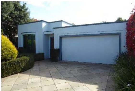
2 Killop Street – façade/south elevation, included in HO362
