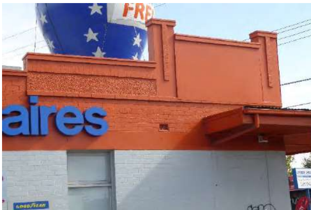
Yarralea Street (east) elevation – parapet detailing
