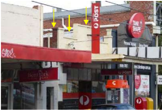
No. 730 – the original parapet, east return and hipped roof are visible from Heidelberg Road
