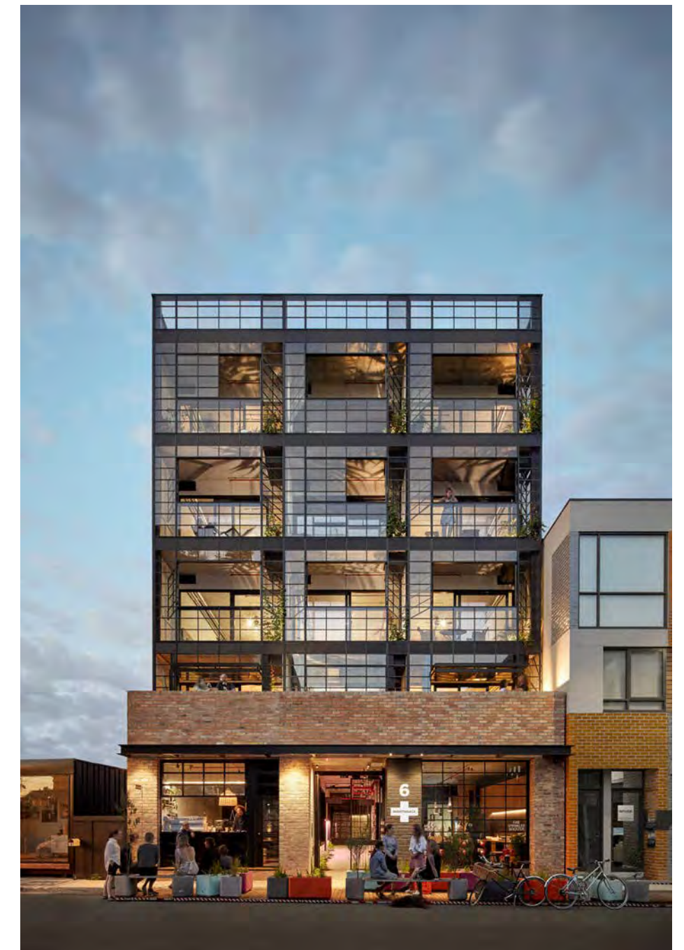
Figure 141. Nightingale 1, Brunswick (Source: Breathe Architecture)
