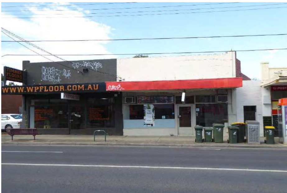
Side access no. 730A (right), no. 732 (centre) and no. 734 (left)
