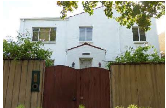
Park Crescent (south elevation) – original openings
