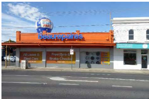
Heidelberg Road (north) elevation
