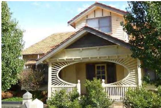
59 Yarralea Street – east elevation, included in HO362
