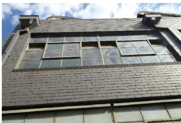
Steel framed windows on the Arthur Street (east) facade
