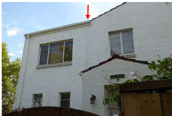
House – Park Crescent (primary) façade Junction between original (right) and additions (left)
