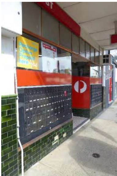
No. 730 Heidelberg Road – typical Interwar shopfront configuration
