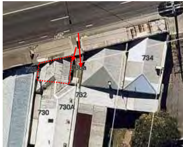
No. 730 – original section of roof visible from Heidelberg Road indicated by the dotted line. Visible parapet returns of nos 730 and 732 indicated by the red arrows (Source: Nearmap)
