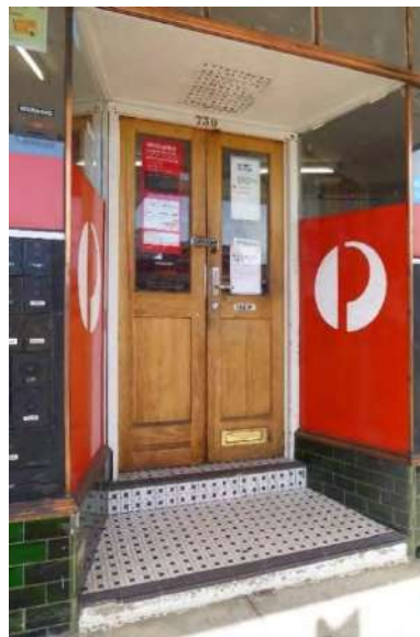
No. 730 Heidelberg Road – recessed entry including original tiles and pressed metal ceiling
