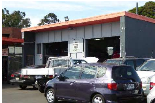
Heidelberg Road - west wing
