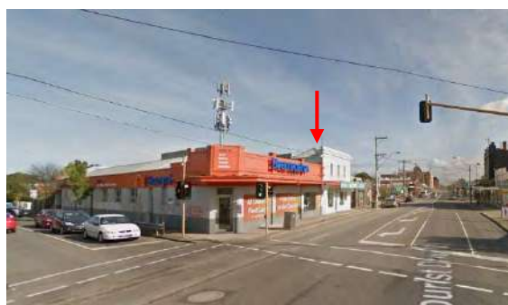
The prominence of the former Butcher Shop (HO71) is evident from the intersection of Heidelberg Road and Yarralea Street (Source: googlemaps)
