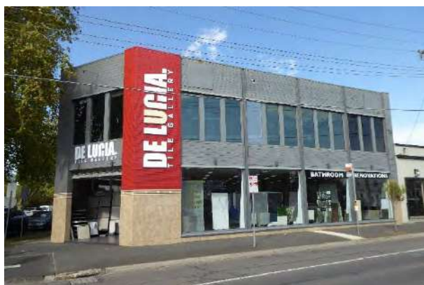
Heidelberg Road (north) elevation
