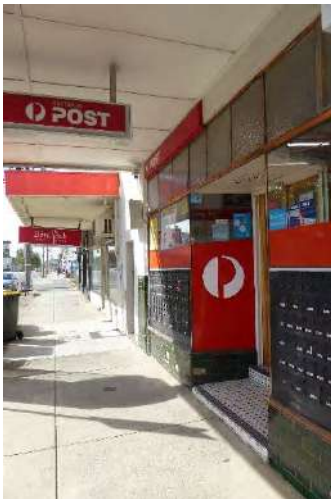
No. 730 – original shopfront
