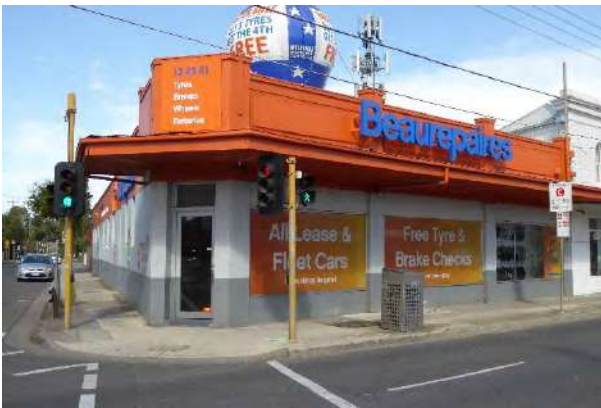
Heidelberg Road (north) elevation
