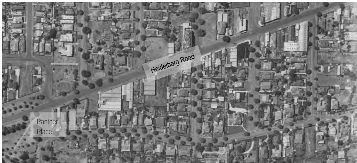
1945 Aerial, Heidelberg Road – west end of study area (between Panther Place and Austin Street) (Source: Landata, Melbourne and Metropolitan Area Project, Proj. No. 5, Run 27, Frame 59,529)
