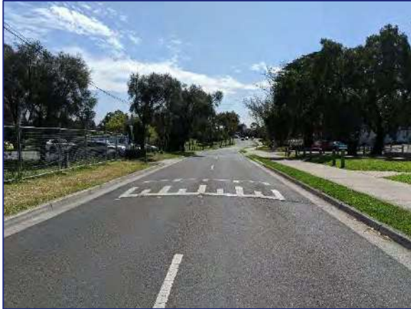
Figure 13: Yarra Bend Road - view north
