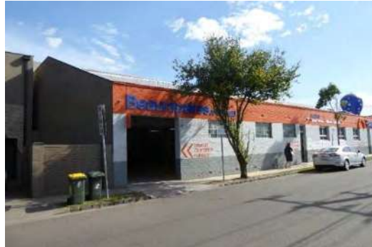
Original roof form and openings along Yarralea Street
