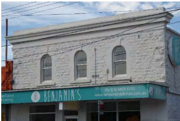
Symmetrical first floor features three original arched windows
