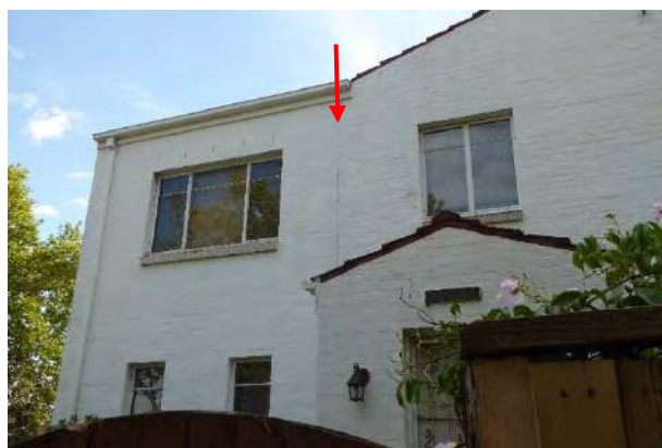
House – south elevation, window openings and portico. The junction between the original eastern section and later west wing is evident.
