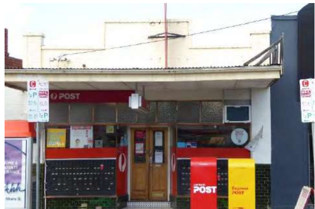
730 Heidelberg Road – parapet and shopfront
