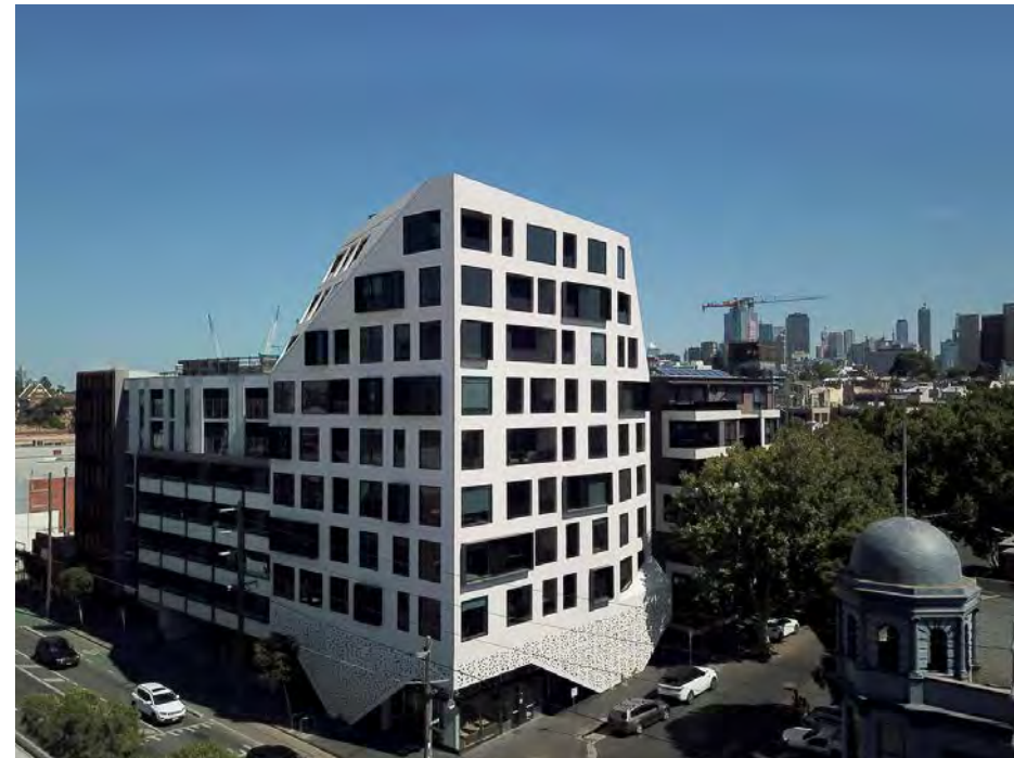
Figure 111. Peel Street, Collingwood [Source: DKO Architecture]
