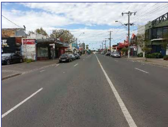
Figure 9: Precinct 3b – Heidelberg Road – view east
