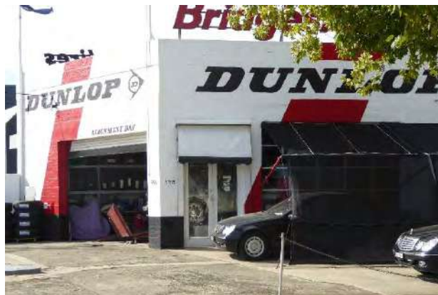
Service centre – west elevation
