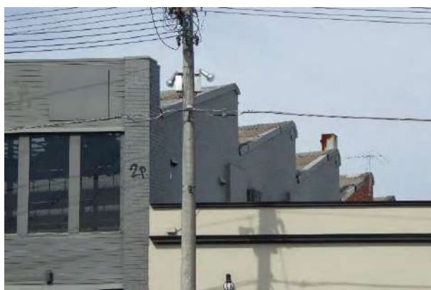
Sawtooth roof forms from Heidelberg Road
