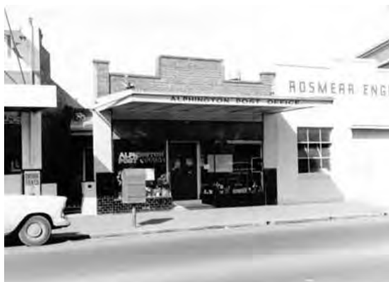
1968 Heidelberg Road elevation – no. 730 (Alphington Post Office) (Source: NAA)
