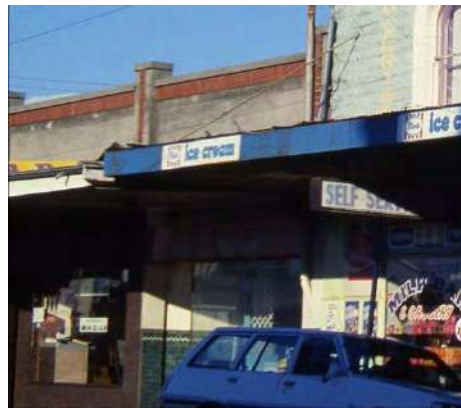
1982 image – showing original parapet detailing
