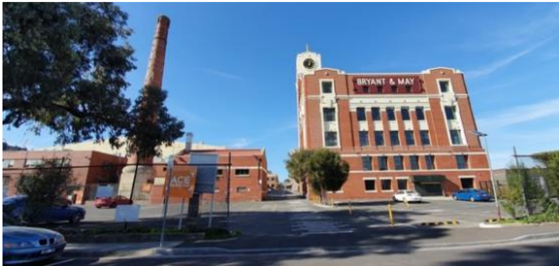
Figure 42. View through the Bryant and May site from the immediate west. Source: Trethowan Architecture.
