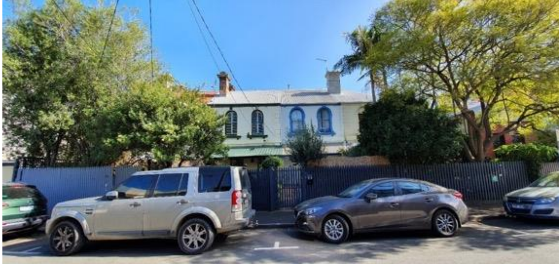
Figure 33. 30-38 Dover Street. Source: Trethowan Architecture.
