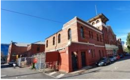
Figure 46. North-western elevation with tower. Source: Trethowan Architecture.
