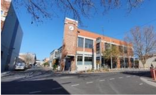
Figure 50. View south into site from Balmain Street to Building 18. Source: Trethowan Architecture.
