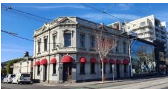
Figure 39. 619 Church Street. Source: Trethowan Architecture.
