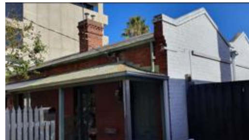
Figure 30. Detail view of the side gables. Source: Trethowan Architecture.
