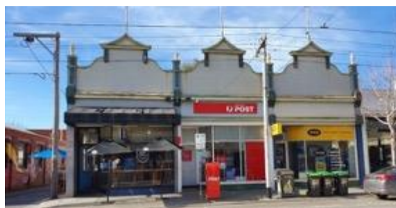
Figure 40. 533-537 Church Street. Source: Trethowan Architecture.
