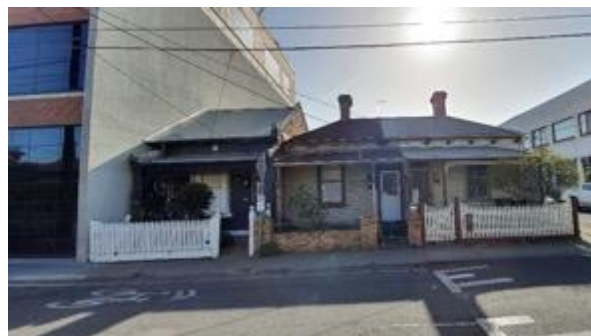
Figure 14. 43-47 Balmain Street showing inappropriate lack of transition between heritage and new development. Source: Trethowan Architecture.
