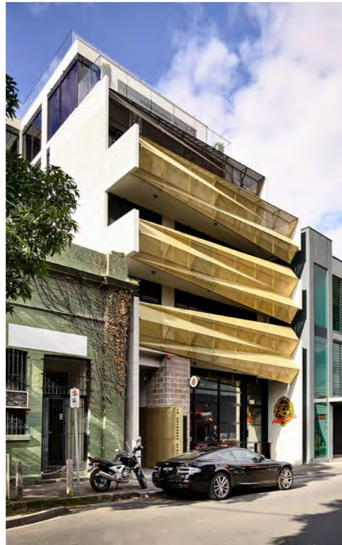
Figure 79. Commercial development in Cremorne (Source: EAT Architects)
