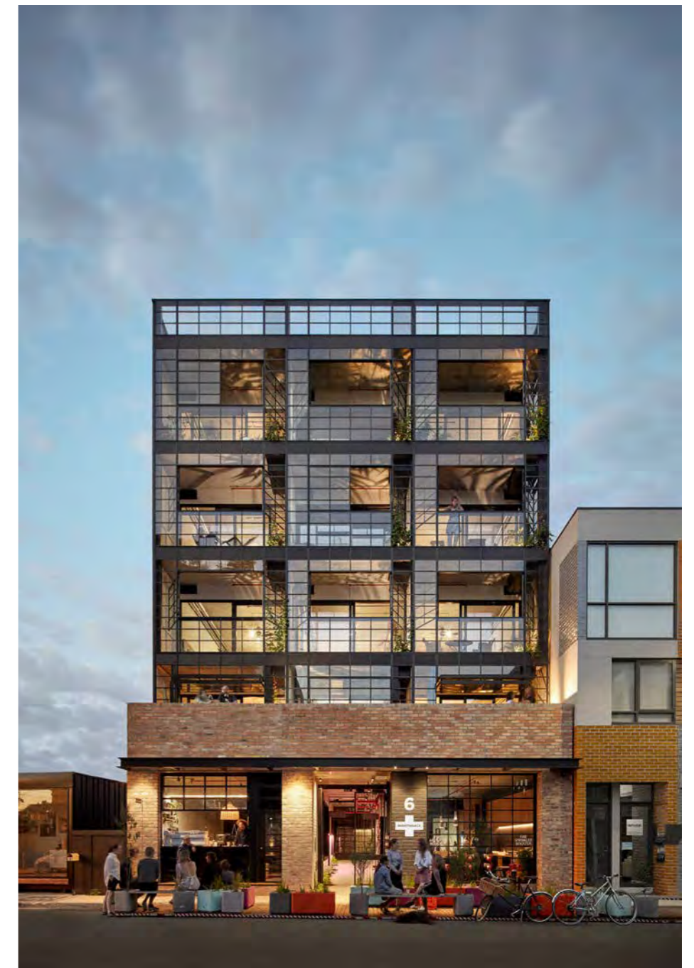
Figure 141. Nightingale 1, Brunswick (Source: Breathe Architecture)
