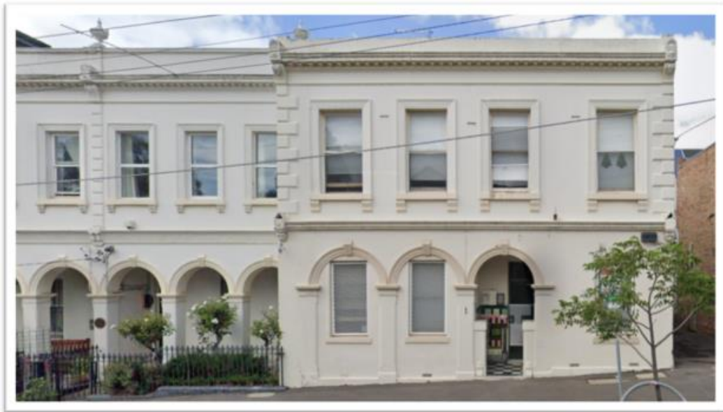
Figure 11: Adjacent dwellings at Nos. 1-7 Derby Street
