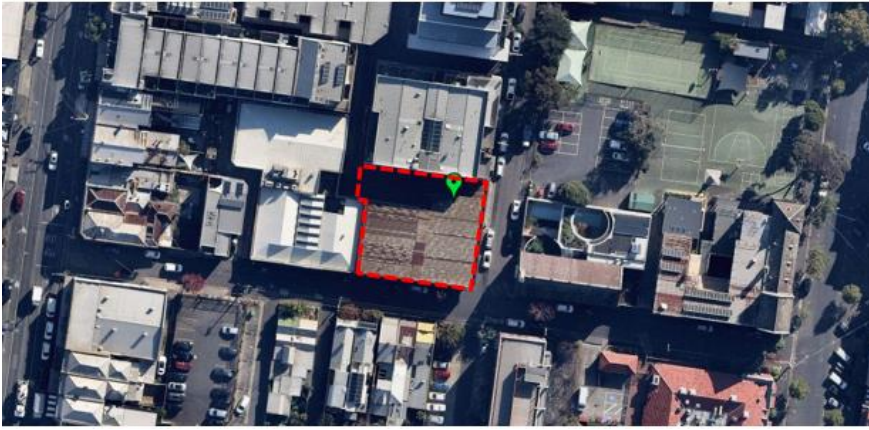
Figure: Aerial photograph of the subject site and surrounding built form Source: Nearmap image capture date: 29 April 2021
