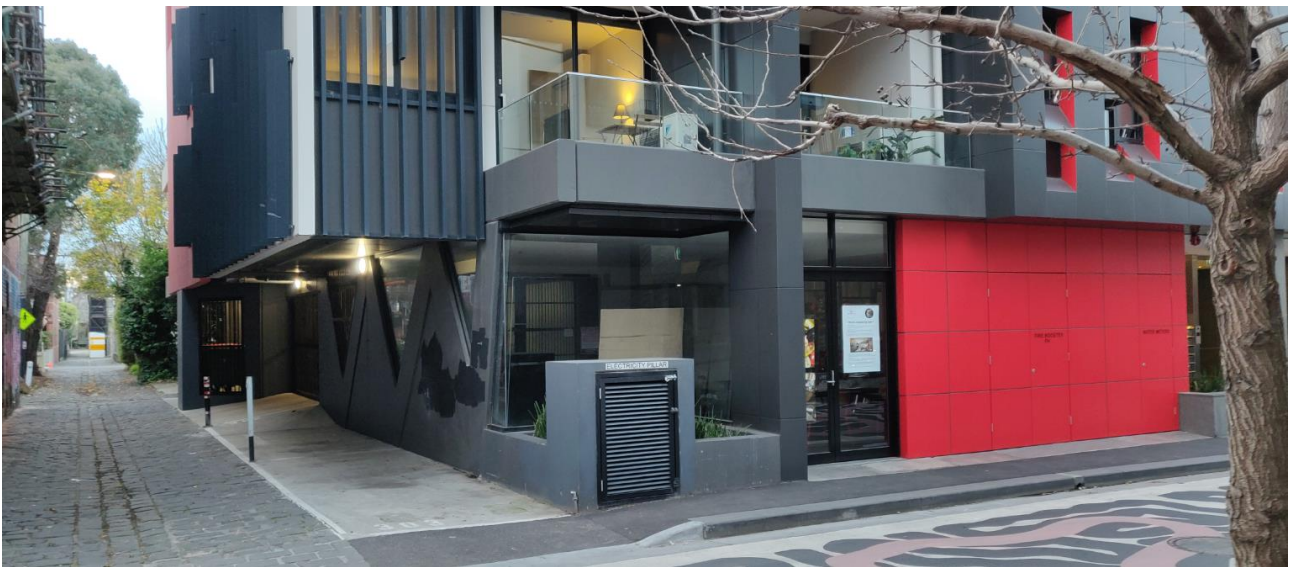
Image 3: Site frontage to Mechanics Lane (Officer Photo, 2021)
