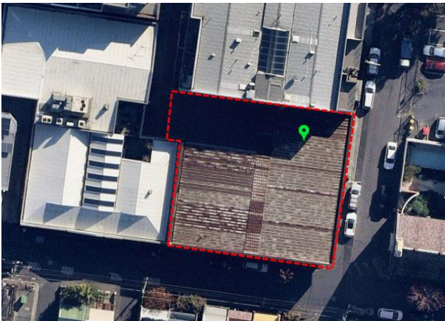
Figure: Aerial photograph of No. 1 – 13 Oxford Street, Collingwood Source: Nearmap, image capture date: 29 April 2021
