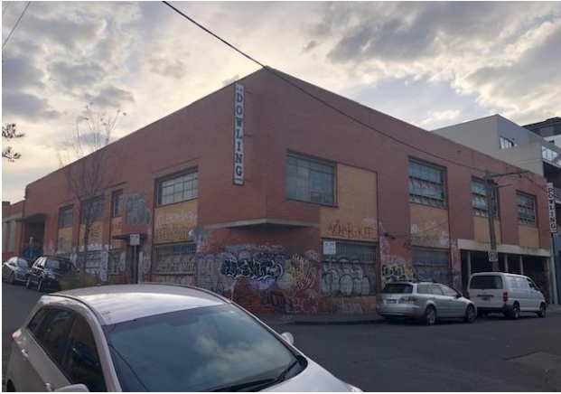
Figure: Subject site at the corner of Oxford and Mason Streets Source: Officer image, taken 21/05/2021
