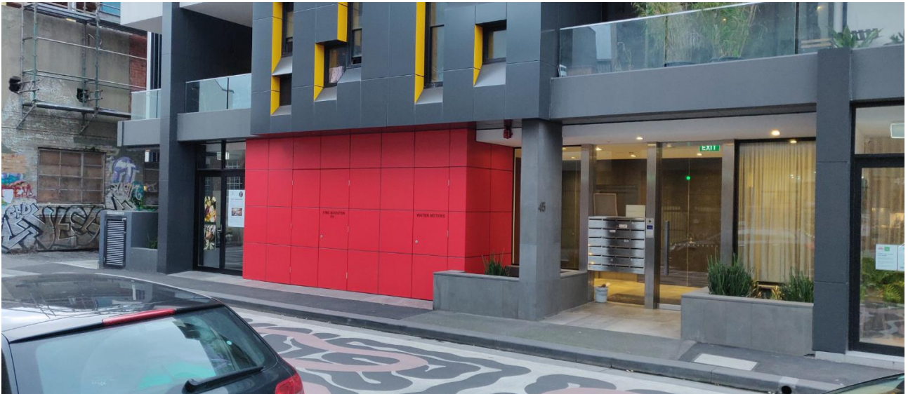
Image 2: Site frontage to Rose Street (Officer Photo, 2021)
