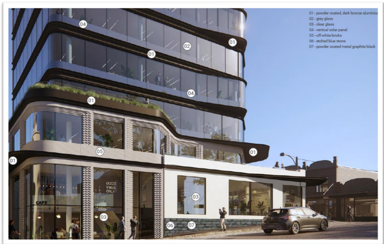
Figure 5: Materials and finishes
