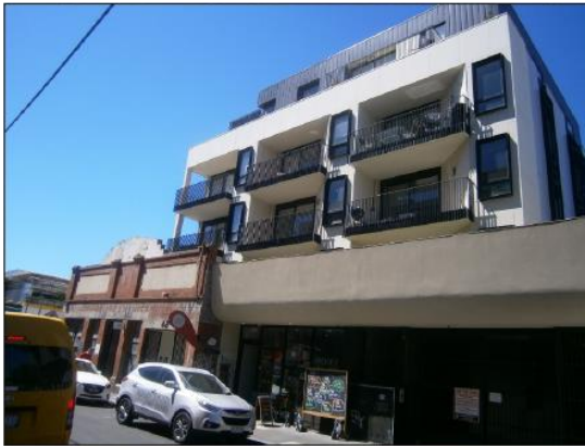
Development opposite the site
