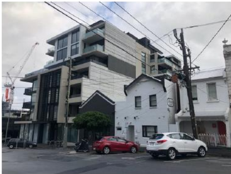
Figure 17: Development at 15-21 Derby Street & 29 Oxford Street (8 storeys, 4-storey street wall), 30m east of the subject site.
