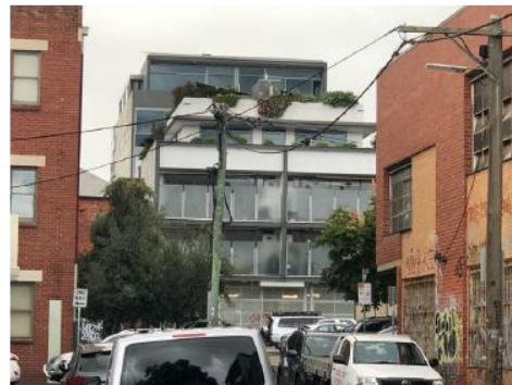
Figure 10: Apartment development fronting Victoria Parade, south of the subject site (at right).
