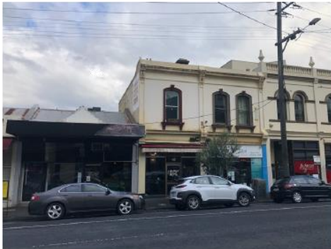
Figure 05: The subject site's southern interface (Smith Street, east side), comprising single-level shop building (left) adjacent to double-storey built form.
