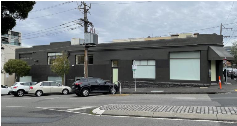
Figure 4 Subject property, northern presentation to Derby Street; showing the long north elevation of 52 Smith Street
