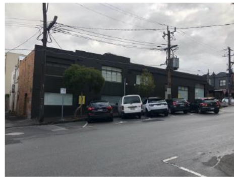
Figure 02: Subject site, Derby Street frontage and rear laneway interface.
