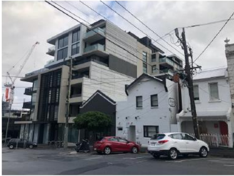
Figure 11: Development at 15-21 Derby Street (8 storeys, 4-storey street wall), 50m east of the subject site.
